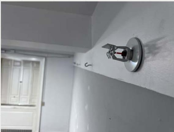
The sprinklers in the studio are horizontally mounted. These sprinklers will be moved and converted to overheads.
