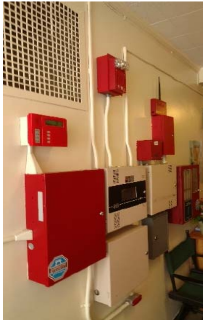
Fire Alarm Control Panels
