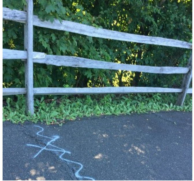
Transverse crack with bump
