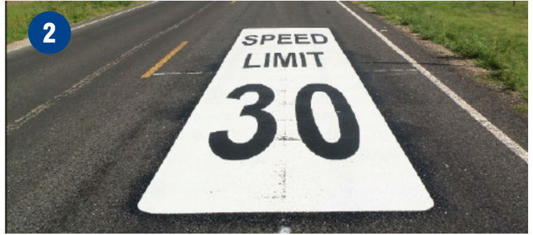
Pavement markings can serve as a traffic calming strategy to advise drivers of the speed limit and/or as they approach areas with high pedestrian or bicycle traffic
