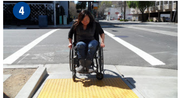
Example of an ADA-compliant curb ramp with a tactile strip
