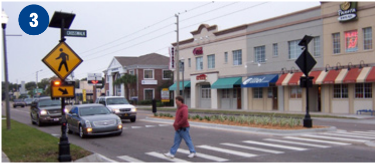
RRFBs enhance safety by increasing pedestrian visibility to drivers approaching unsignalized intersections and mid-block crossings
