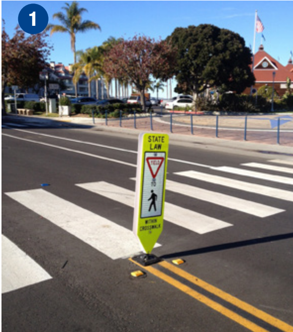
In-street pedestrian signs are installed on bollards located on the centerline to serve as a visible reminder to drivers
