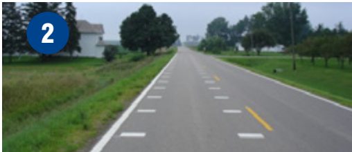
Pavement markings can be used to calm traffic. One study found that converging chevron pattern pavement markings reduced speeds by 5 MPH in mean speeds and by 7 MPH in 85 th percentile speeds. Another study found that transverse pavement marking decreased speeds by 2 MPH in mean and 85th percentile speeds.
