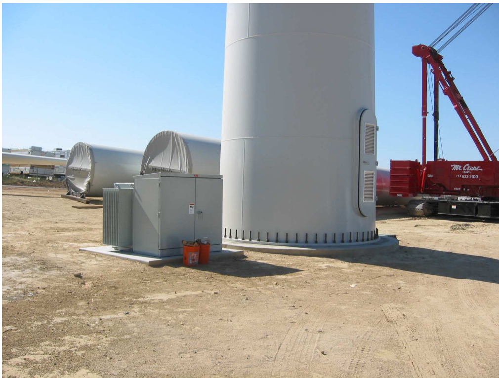
Figure 3-16 Typical Wind Turbine Transformer Arrangement
