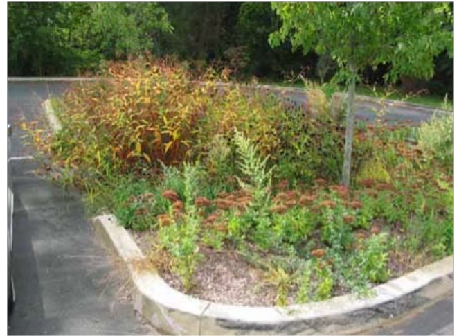
Parking Lot Island Configured as Bioretention (CT DEP LID Appendix)
