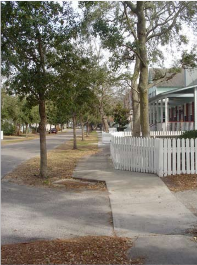
Runoff From Impervious Paved Surfaces Directed to Vegetated Areas (Image: Josh Martin)
