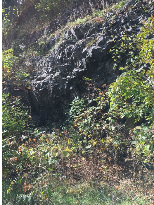
Photo 1 – Rock Slope No. 1: 65-75° dip inclined into slope, creating overhang.
