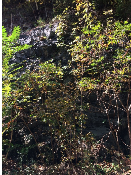
Photo 6 – Rock Slope No. 2: Slope is covered in thick vines and trees up to 10 in. diam.
