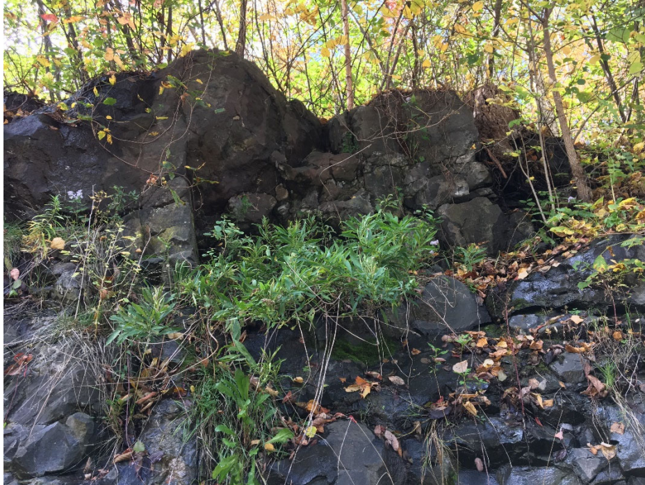
Photo 8 – Rock Slope No. 3 South: Scarp with large blocks at top of slope.
