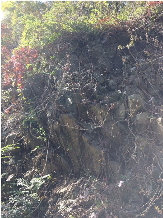
Photo 1 – Rock Slope No. 1: 65-75° dip inclined into slope, creating overhang.
