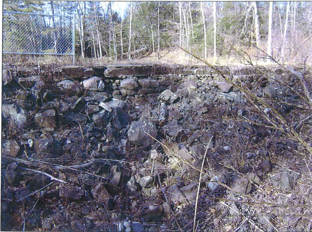
Photo 4: Left side of embankment, with dumped riprap repair
