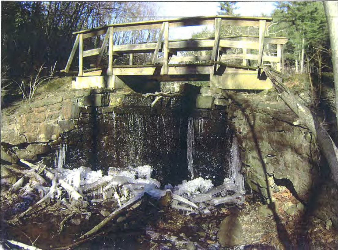
Photo 4: Main spillway and wing walls
