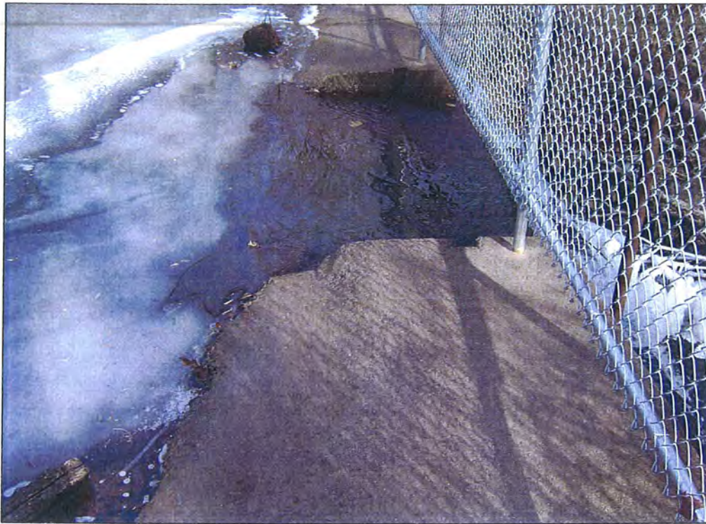
Photo 6: Spillway - cast into concrete cap
