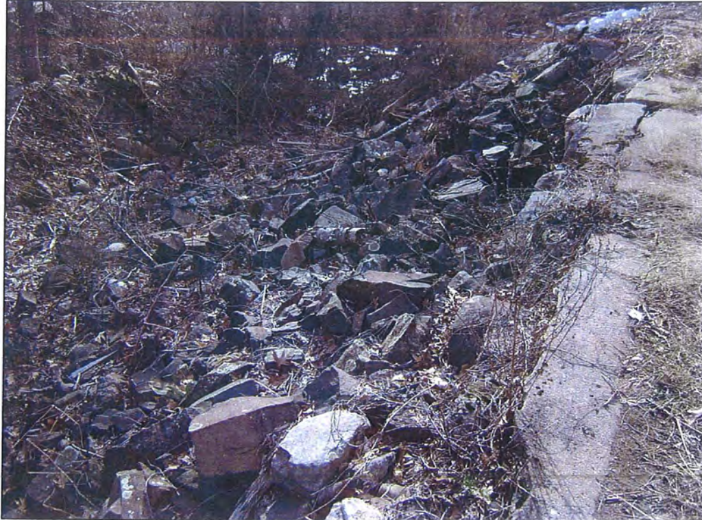
Photo 14: Riprap repair downstream left
