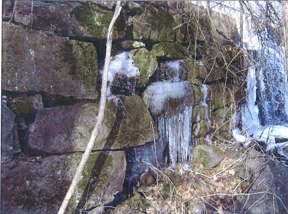
Photo 2: Leak in rubble embankment
