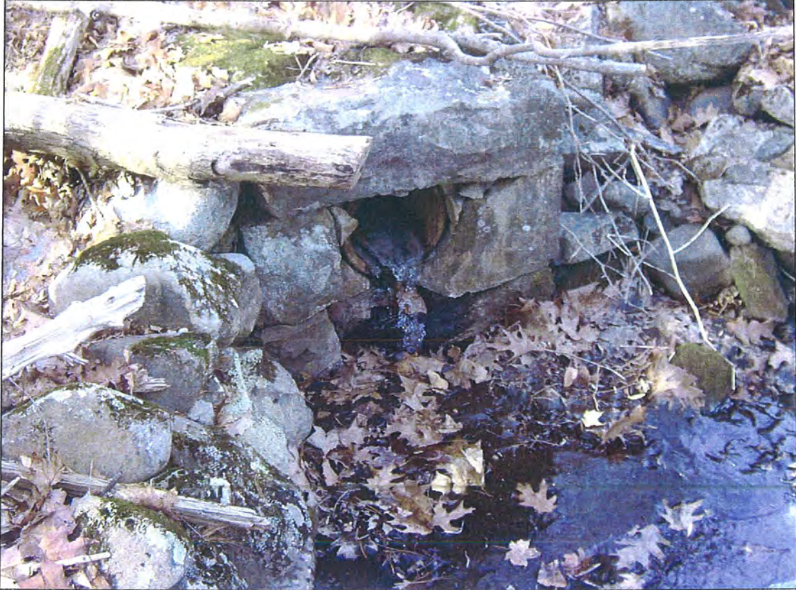
Photo 11: Pipe Outlet with rubble masonry endwall
