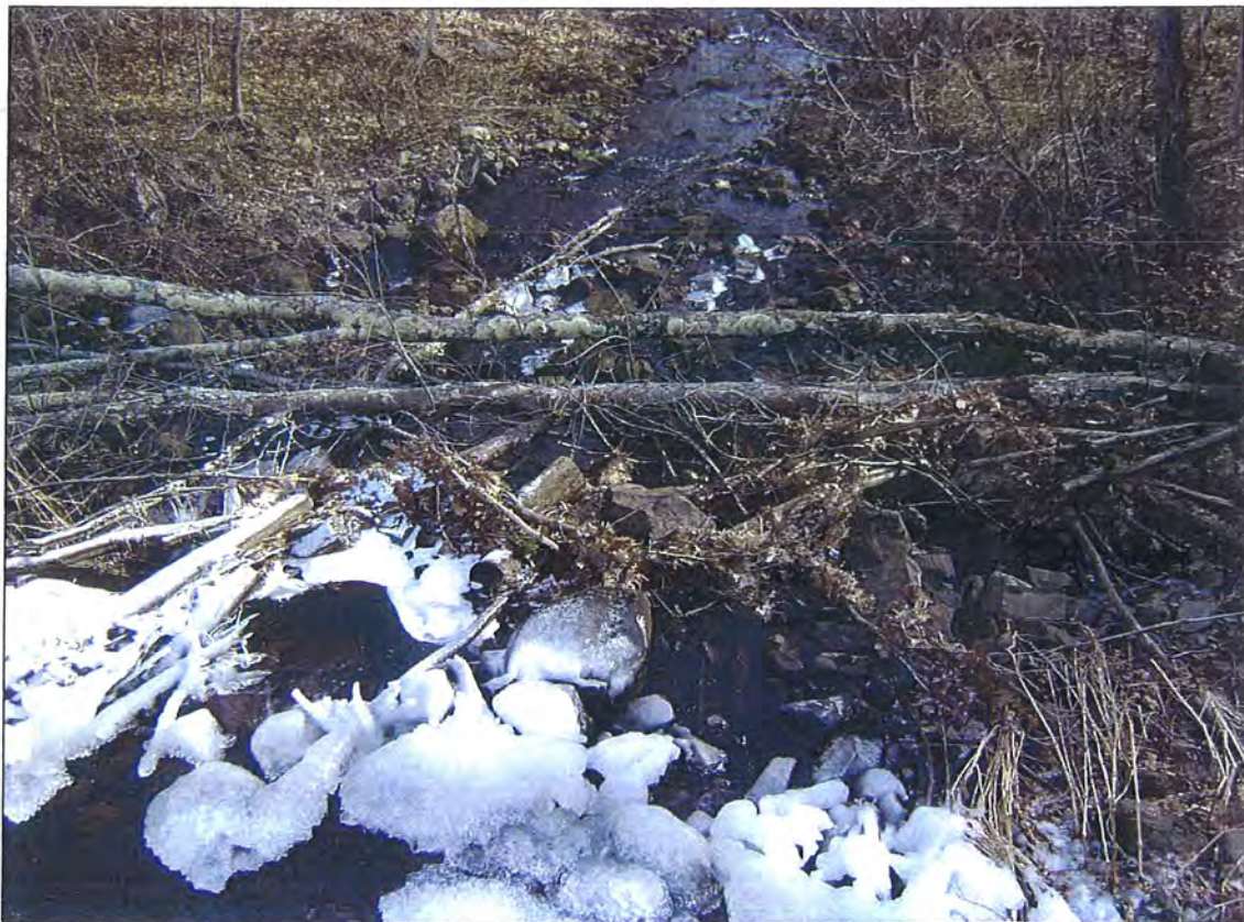
Photo 8: Debris in outlet channel just downstream of spillway
