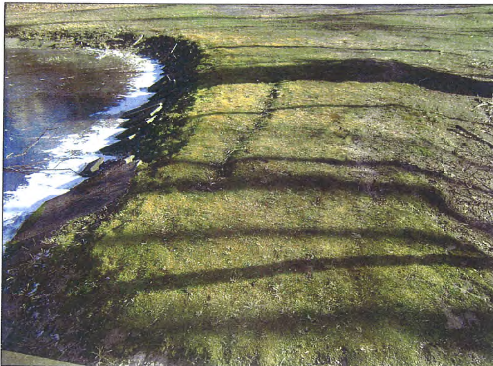
Photo 3: Left abutment, ruts on embankment, concrete paver protection
