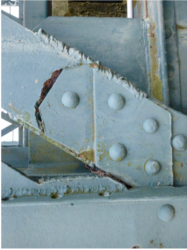
Photo # 28: North elevation of North Truss diagonal member L6-U5 at L6. Note the section loss and rust hole at the connection plates (typical). Also, note the repair plates and retrofitted gusset plate.
