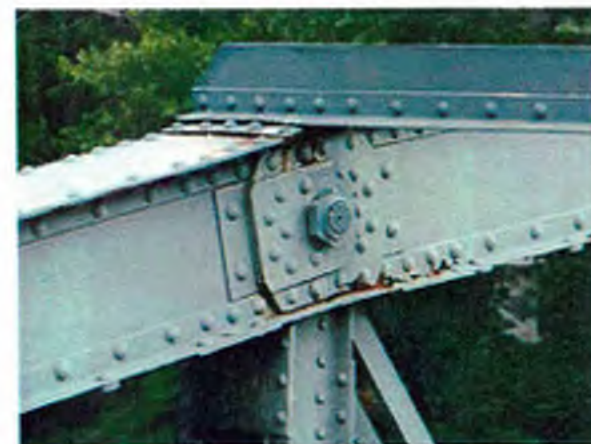
Photo 6 -Spot corrosion at truss connection.
