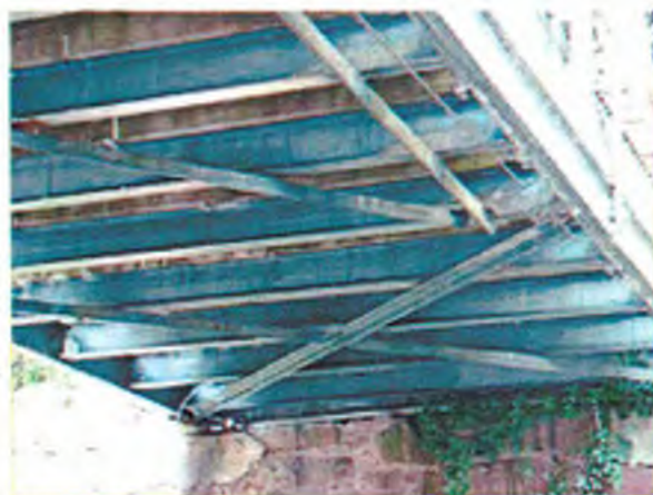
Photo 13 – Typical condition of floor beams.
