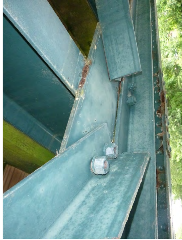
Photo # 35: Bottom lateral bracing connection near L7 in North Truss. Note the short bolts.
