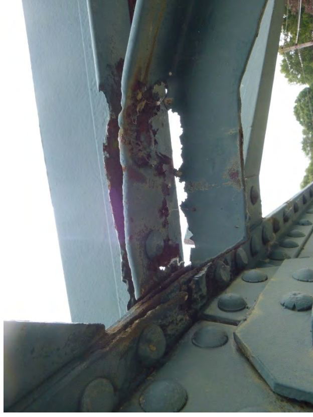
Photo # 38: Sway bracing at U7 above North Truss. Note the section loss with rust holes.
