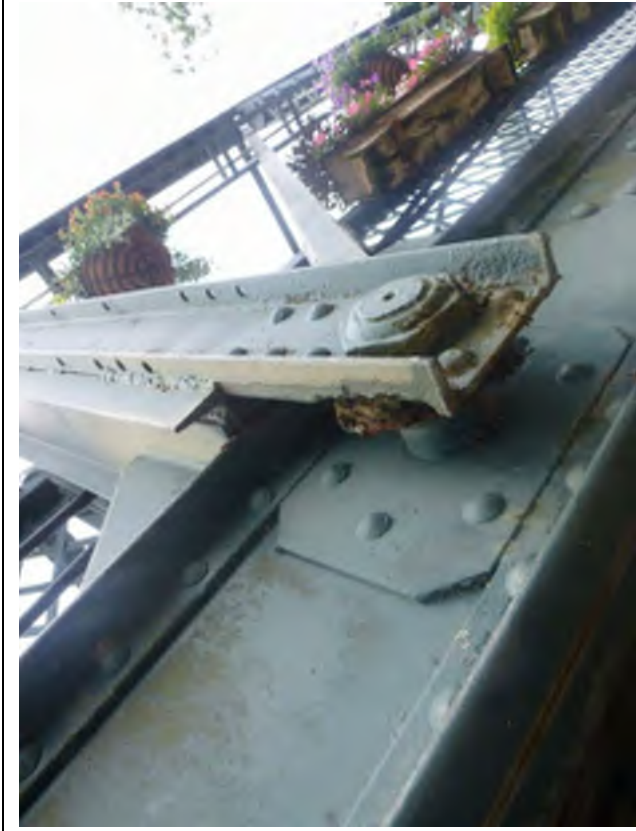
Photo # 23: Exterior view of bottom chord at L3 in North Truss. Note the deterioration along the pin connection.
