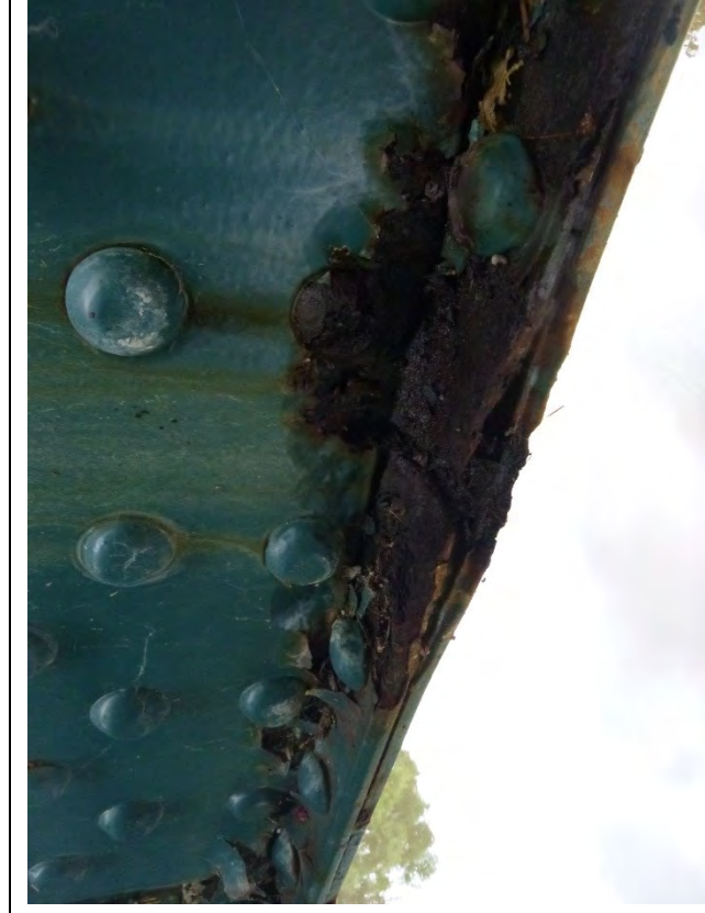
Photo # 25: Pack rust and section loss at the bottom chord splice connection between L2 & L3 in South Truss.
