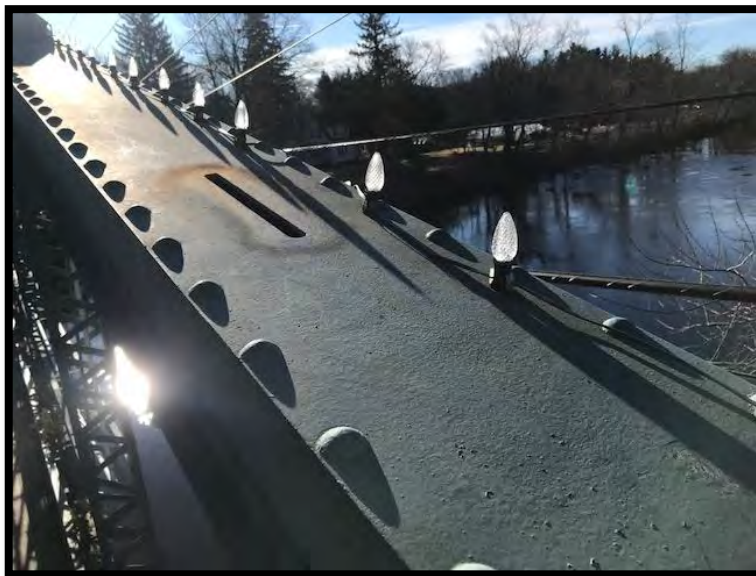
Photo 3: Top plate of top chord after coupon extraction.
