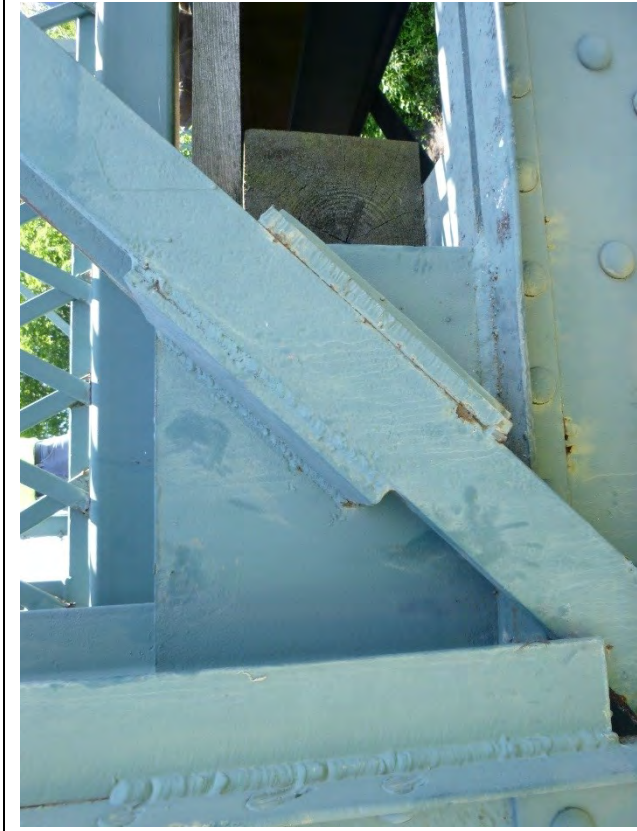
Photo # 31: South elevation of typical repair for eye bar at L10 in South Truss.
