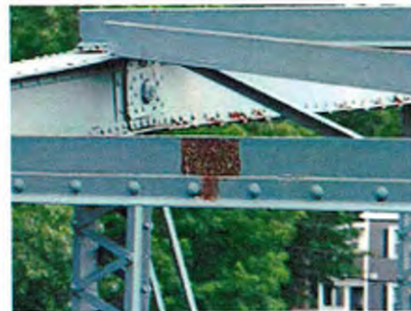
Photo 7 -Spot corrosion on truss bracing.
