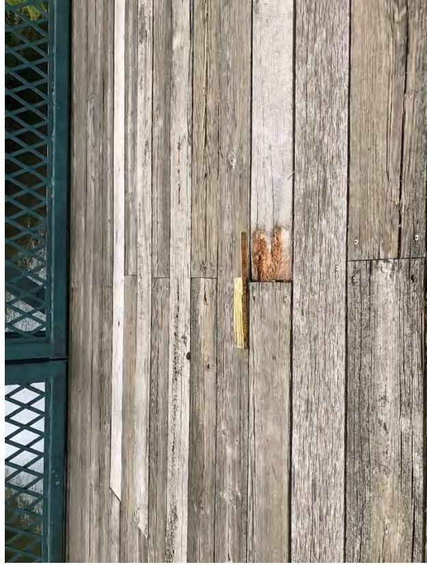
Photo # 8: Isolated timber rot in the deck near midspan with exposed nails.
