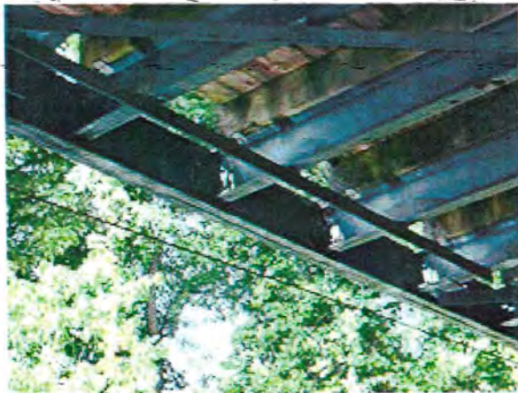
Photo 14 – Typical condition of floor beams.
