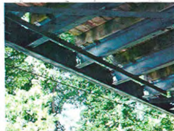
Photo 14 – Typical condition of floor beams.
