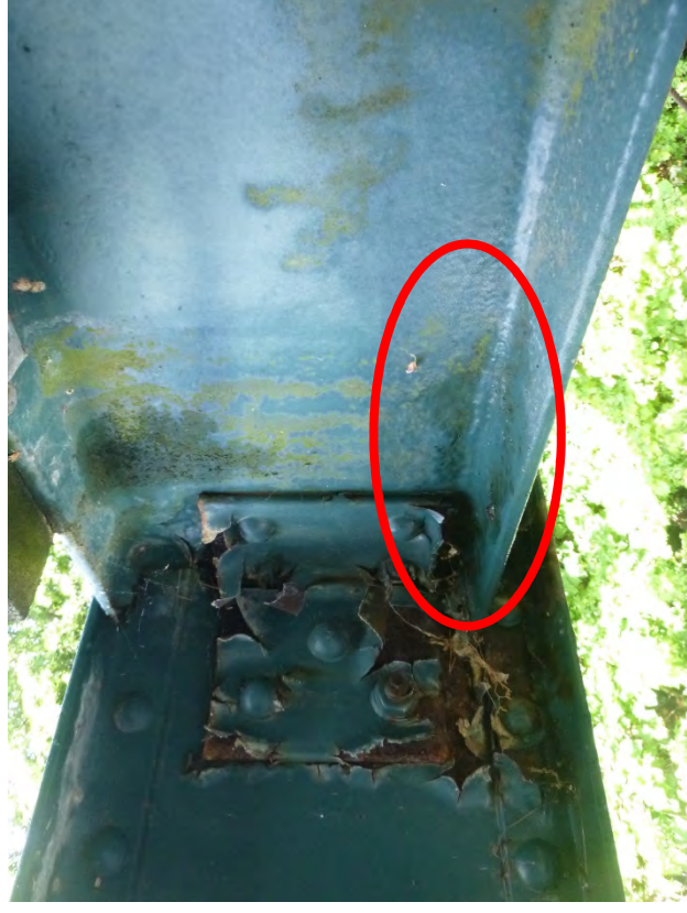
Photo # 20: Clip angle at Floorbeam FB2 between L1 & L2. Note peeling paint with rust. Also, note the painted over pitting along the bottom of floorbeam web.
