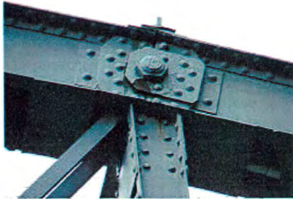
Photo 3 –Spot corrosion on truss connection.
