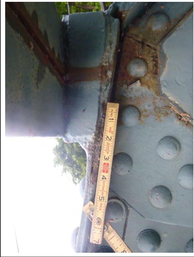
Photo # 39: North side of U1 in South Truss. Note the crack in the weld.
