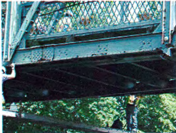
Photo 8 – Spot corrosion on truss lower chord.
