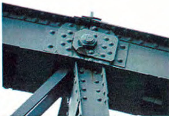
Photo 3 -Spot corrosion on truss connection.
