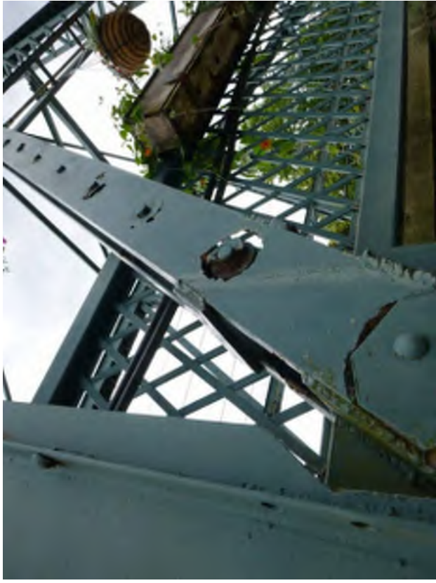
Photo # 30: North elevation of North Truss diagonal member L6-U5 at L6. Note the section loss with rust holes in the channel web.
