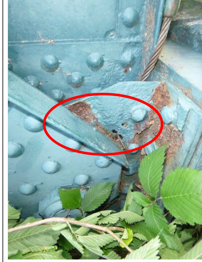
Photo # 17: Fixed bearing for North Truss at East Abutment. Note the section loss with rust holes.
