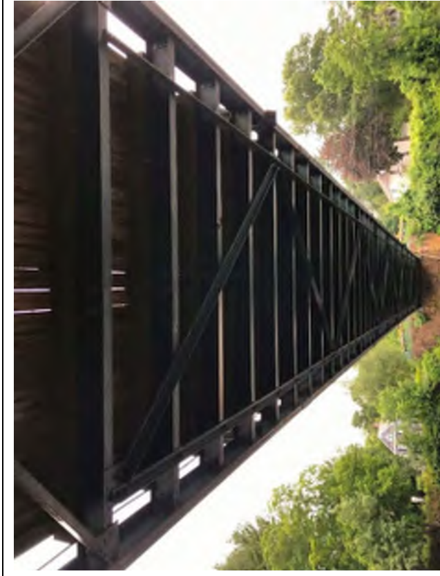
Photo # 9: View of the underside of deck and framing. Note the gaps between the deck planks.
