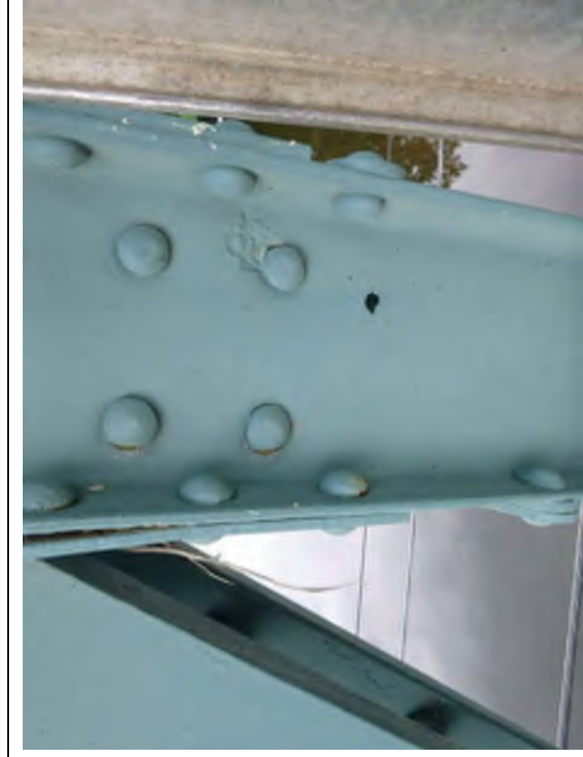
Photo # 27: Vertical member in U5 South Truss. Note the rust hole.
