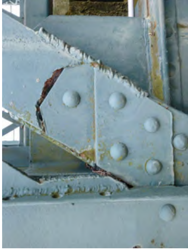
Photo # 28: North elevation of North Truss diagonal member L6-U5 at L6. Note the section loss and rust hole at the connection plates (typical). Also, note the repair plates and retrofit gusset plate.
