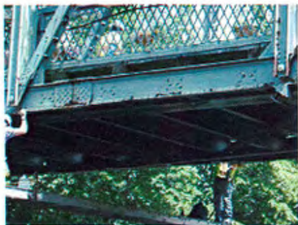
Photo 8 – Spot corrosion on truss lower chord.
