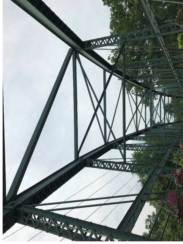
Photo # 36: View of the top strut, sway bracing and lateral bracing between north and south trusses.
