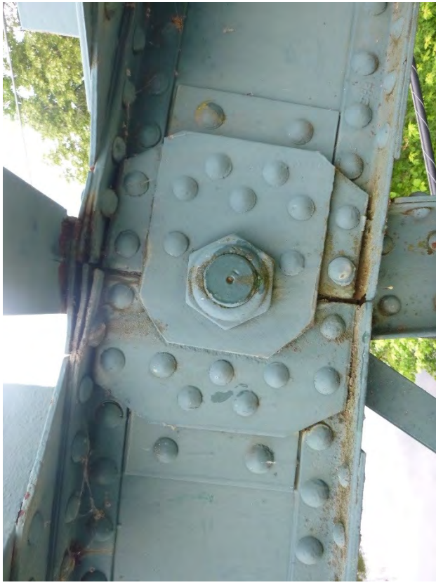
Photo # 32: North elevation of top chord member in South Truss at U2. Note the bent down top angles at the connection due to pack rust (typical).
