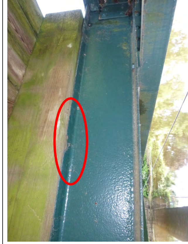
Photo # 19: Floorbeam FB3 between L1 & L2 in South Truss. Note the section loss with rust hole in top flange of the floorbeam.
