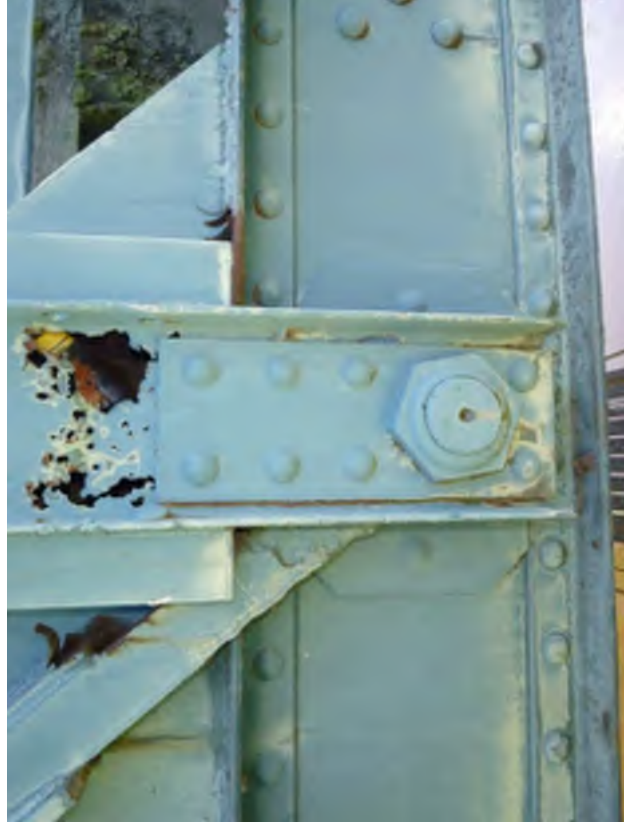
Photo # 26: South elevation of vertical member in South Truss at L3. Note the section loss in the diagonal eye bar and web of truss vertical member. Also, note the repair plates and channel atop the bottom chord.
