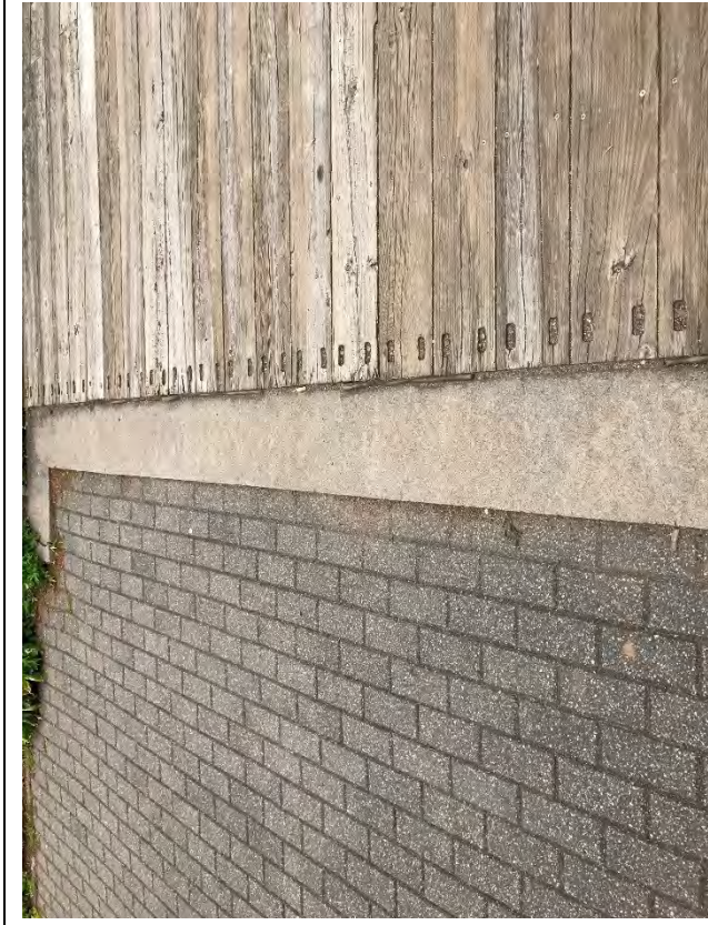
Photo # 13: Deck end joint at West Abutment. Note the deteriorating joint sealant material.
