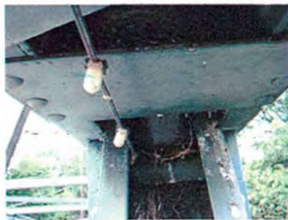
Photo 5 -Bird nest in truss top chord.
