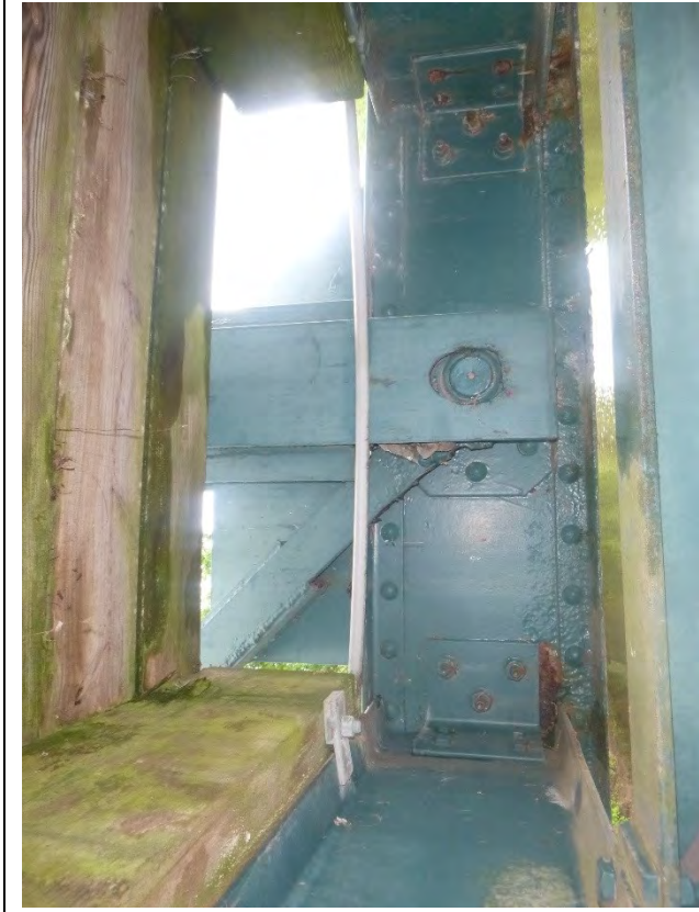
Photo # 21: Interior view of the bottom chord at L2 in North Truss. Note the deterioration along the pin connection and the repair plates.
