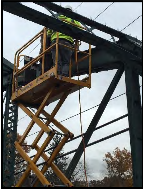
Photo 1: Coupons extraction operations
