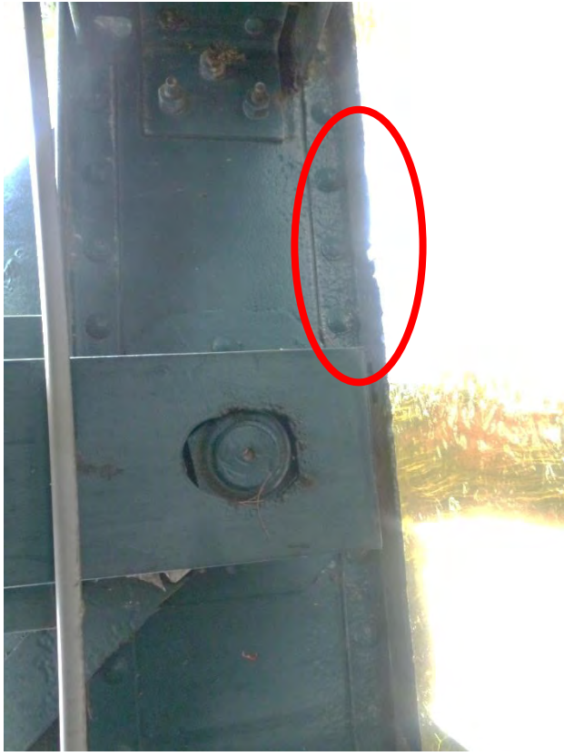
Photo # 22: Interior view of the bottom chord at L2 in North Truss. Note the pitting along the interior bottom angle.
