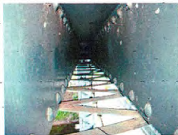
Photo 4 -Typical view of interior truss top chord.
