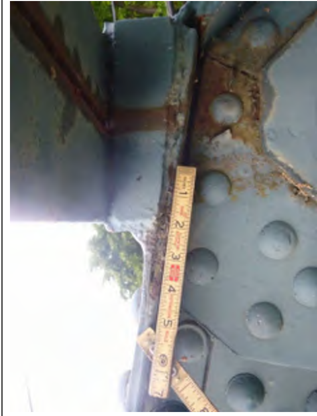
Photo # 39: North side of U1 in South Truss. Note the crack in the weld.
