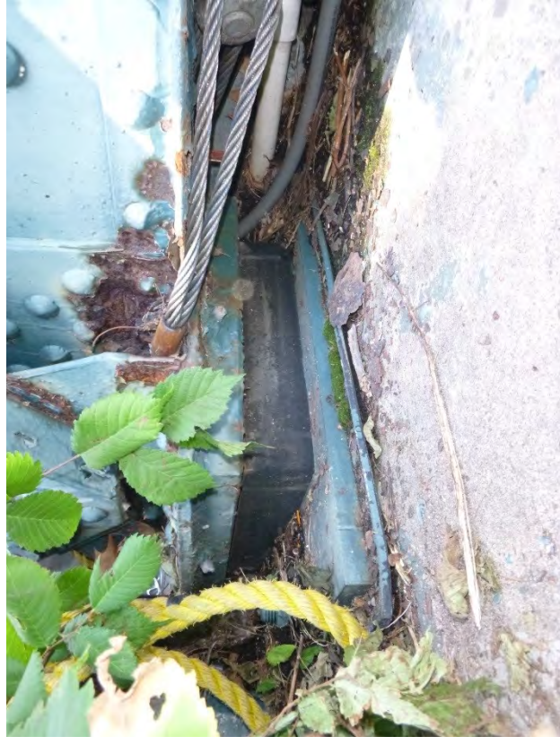
Photo # 16: Expansion bearing for South Truss at West Abutment.
