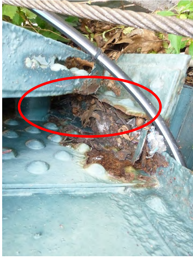
Photo # 18: Expansion bearing for North Truss at West Abutment. Note the missing gusset plate. Also, note the rust hole in horizontal leg of top chord bottom angle.
