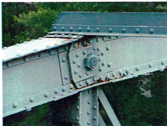
Photo 6 –Spot corrosion at truss connection.
