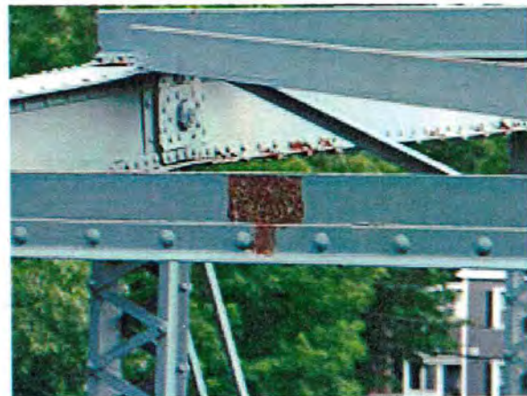
Photo 7 –Spot corrosion on truss bracing.
