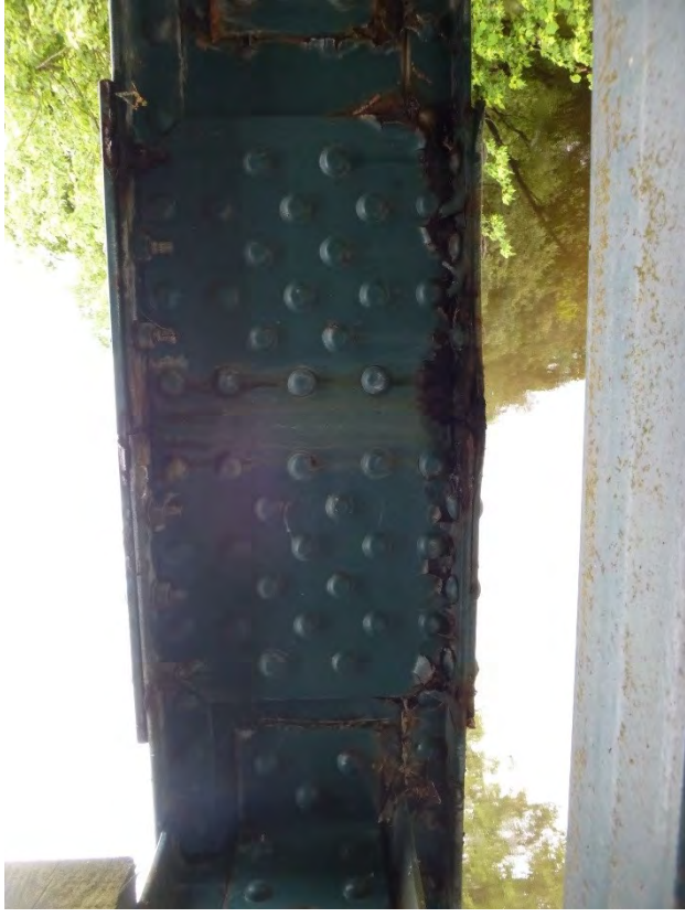
Photo # 24: Bottom chord splice connection between L2 & L3 in South Truss.
