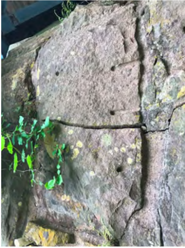
Photo # 44: Crack in the stone masonry at Northeast Wingwall.
