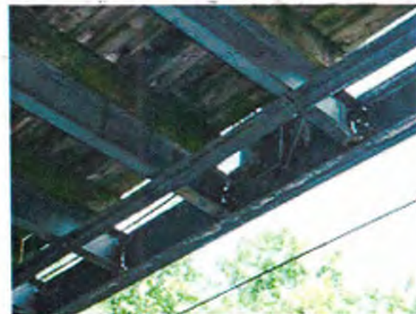
Photo 15 – Typical condition of floor beams.
