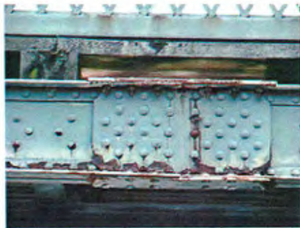
Photo 9 – Spot corrosion on truss lower chord.
