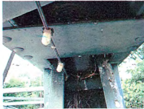
Photo 5 –Bird nest in truss top chord.
