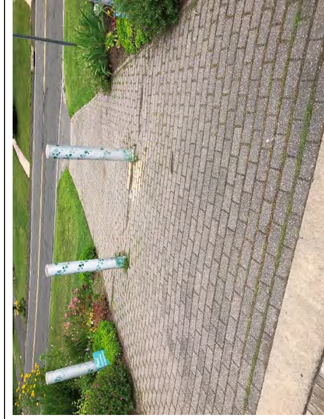
Photo # 15: East approach pavement. Note the depressed area.
