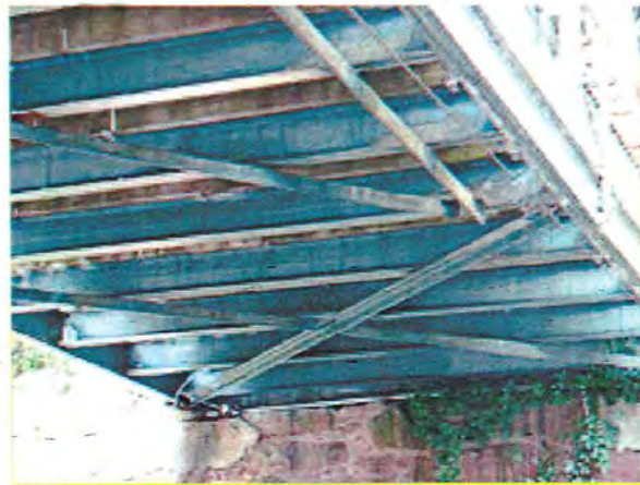
Photo 13 – Typical condition of floor beams.
