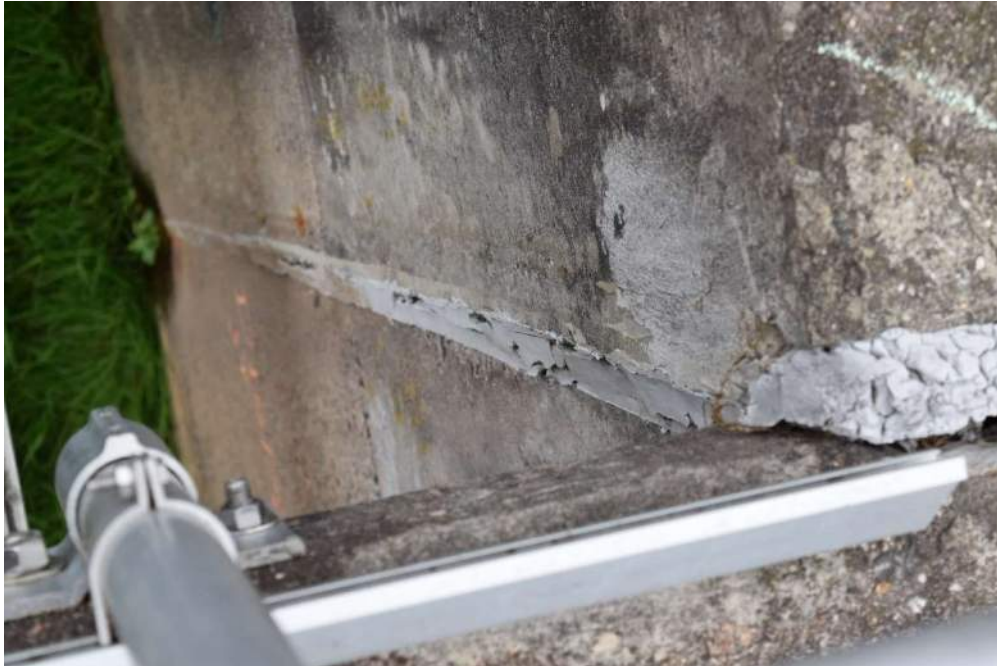
Photo 27 – Expansion Joint at South Wall of Basin No. 2
