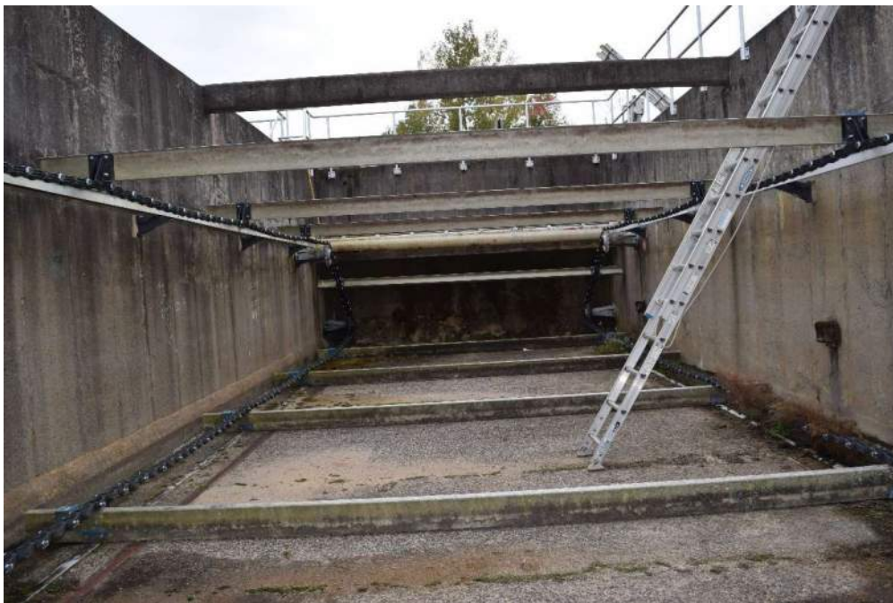
Photo 32 – Center Wall of Basin No. 2 at East Bracing Strut – (Looking North) General view of the connection between the East Strut and the Center Wall of Basin No. 2. Slight cracking was observed at the connection of the strut to the wall.
