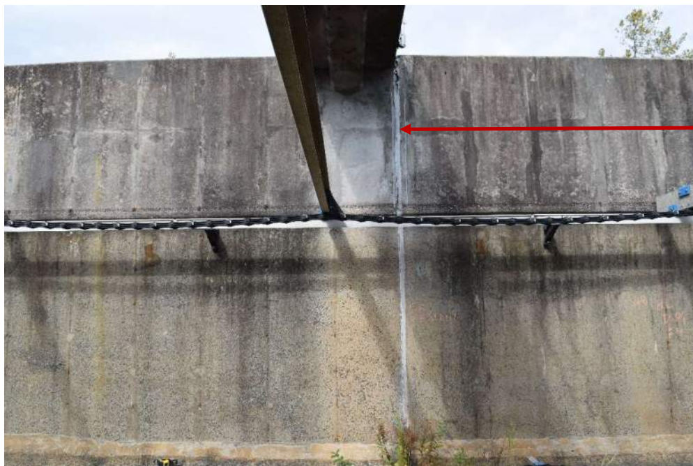
Photo 30 – Center Wall of Basin No. 2 at Center Bracing Strut/Catwalk – (Looking North) General view of the connection between the Center Strut and the Center Wall of Basin No. 2 showing failed Expansion Joint Sealer.
