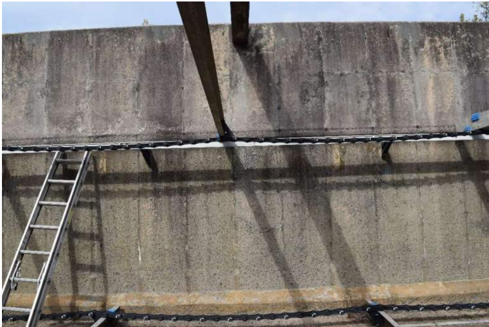
Photo 29 – Center Wall of Basin No. 2 at West Bracing Strut – (Looking North) General view of the connection between the West Strut and the Center Wall of Basin No. 2. Slight cracking was observed at the connection of the strut to the wall.
