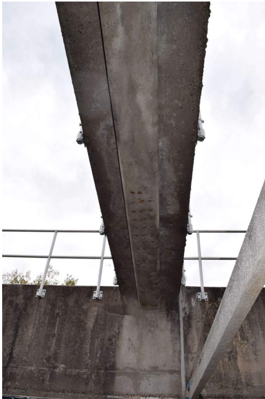
Photo 40 – Underside of Center Strut/Catwalk – Basin No. 1 – (At connection with North Wall) View of exposed reinforcement on the underside of the Center Strut/Catwalk above Basin No. 1.
