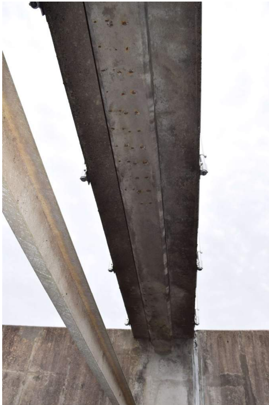
Photo 31 – Underside of Center Strut/Catwalk – Basin No. 2 – (At connection with Center Wall) View of exposed reinforcement on the underside of the Center Strut/Catwalk above Basin No. 2.
