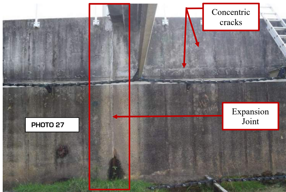
Photo 26 – South Wall of Basin No. 2 at Center Bracing Strut/Catwalk – (Looking South) Connection of the Center Bracing Strut/Catwalk to the South Wall of Basin No. 2. Concentric cracking is visible around the strut on the west side of the Expansion Joint, where the wall is restrained by the strut. On the east side of the Expansion Joint, the wall is unrestrained at the top, and has displaced inward approximately 1 inch.
