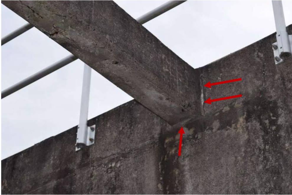
Photo 38 – Connection of North Wall of Basin No. 1 to West Bracing Strut Punching shear cracks along the perimeter of the bracing strut.
