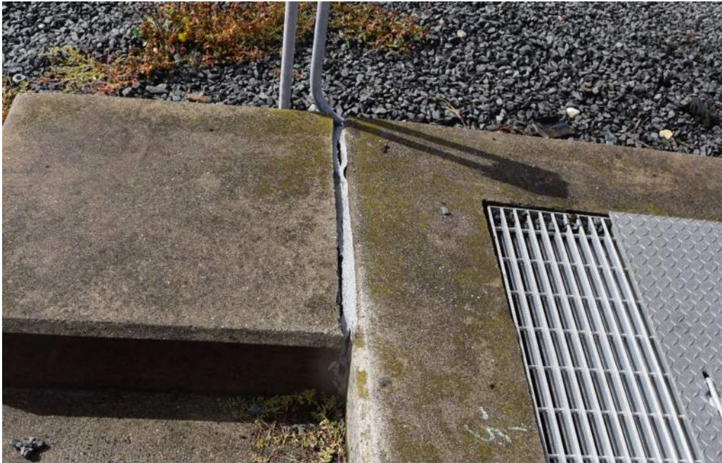
Photo 2 – Cracked Joint Sealant
