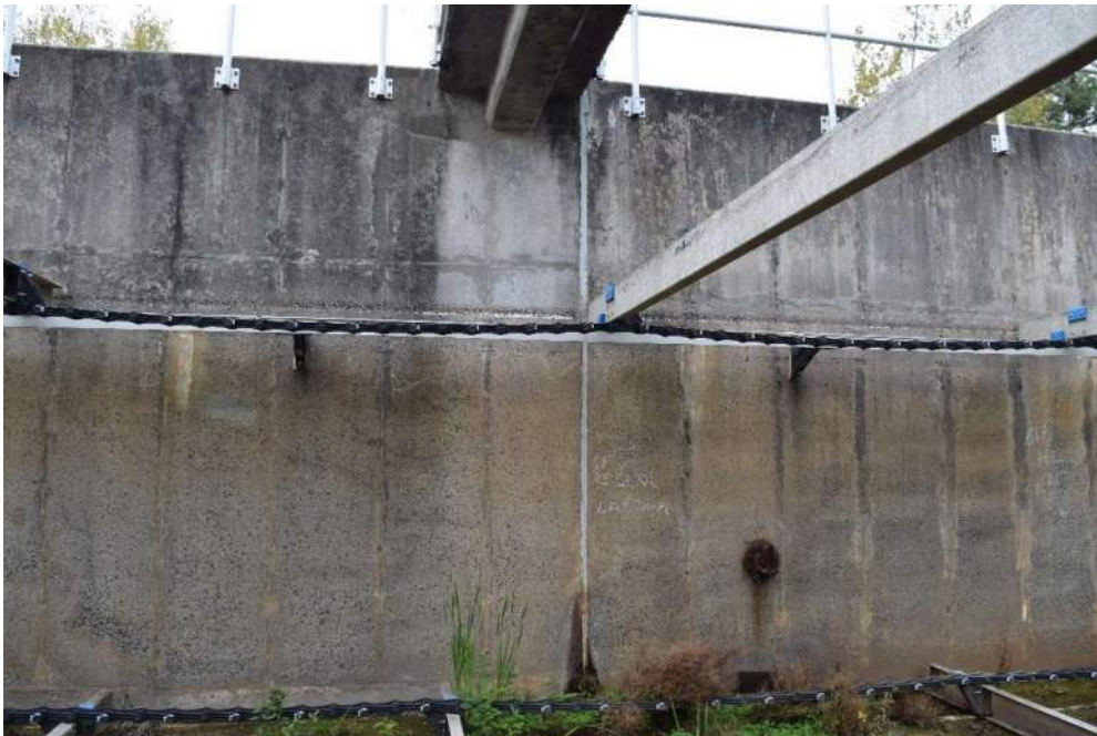
Photo 39 – North Wall of Basin No. 1 at Center Bracing Strut/Catwalk – (Looking North) General view of the connection between the Center Bracing Strut/Catwalk and the North Wall of Basin No. 1.
