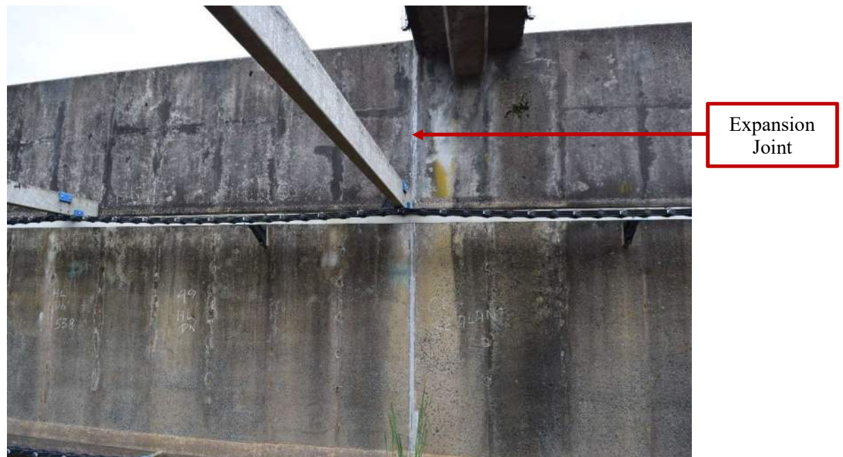
Photo 35 – Center Wall of Basin No. 1 at Center Bracing Strut/Catwalk – (Looking South) General view of the connection between the Center Strut and the Center Wall of Basin No. 2 showing failed Expansion Joint Sealer.
