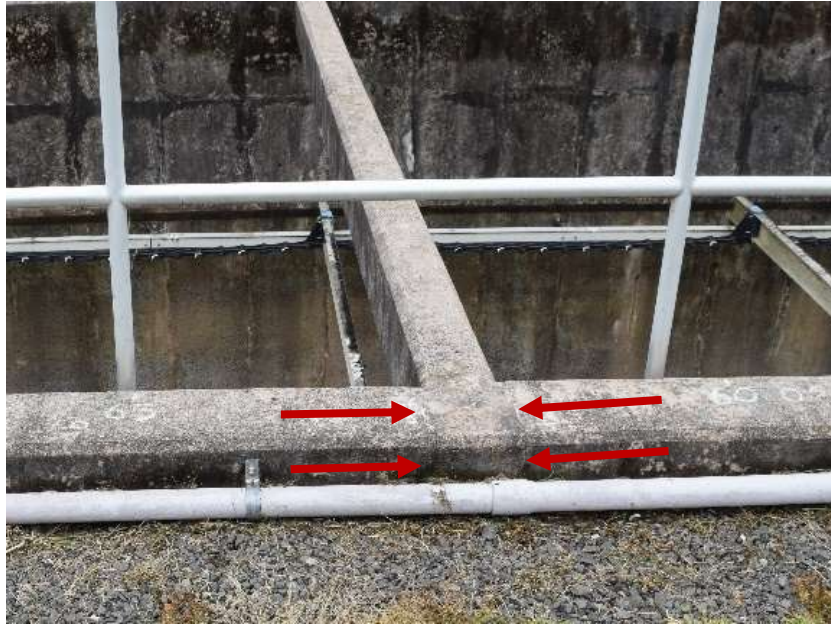
Photo 19 – North Wall of Basin No. 1 at East Bracing Strut (Looking South) Punching shear cracks along the perimeter of the Bracing Strut.
