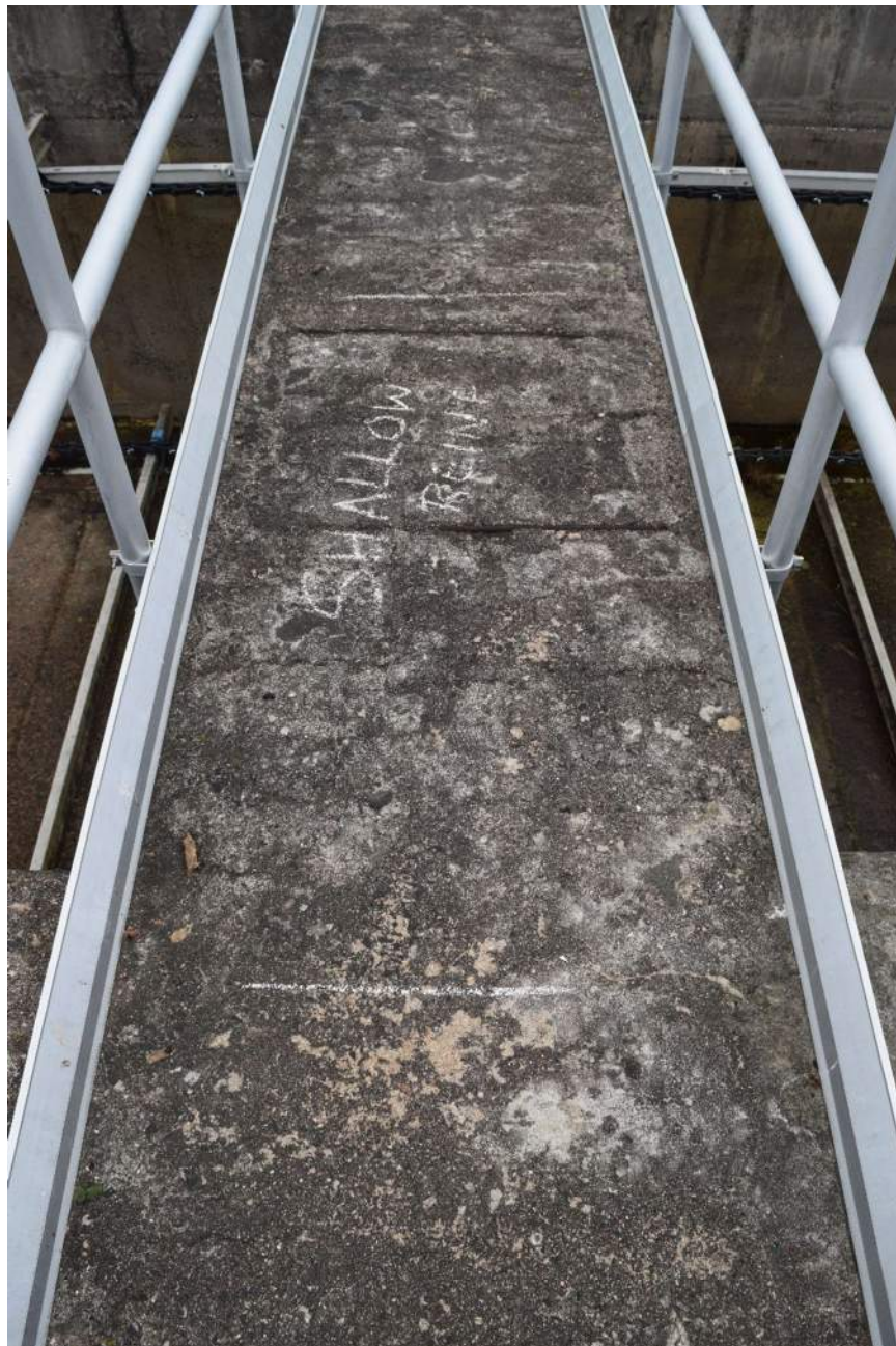
Photo 10 – Center Bracing Strut/Catwalk (Looking North) View of exposed shallow reinforcement at the top of the Center Bracing Strut/Catwalk.
