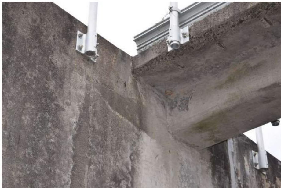
Photo 42 – North Wall of Basin No. 1 at Center Bracing Strut/Catwalk Connection of the Center Bracing Strut/Catwalk to the North Wall of Basin No. 1. Concentric hairline cracking is visible around the strut on the west side of the Expansion Joint, where the wall is restrained by the strut. On the east side of the Expansion Joint, the wall is unrestrained at the top, and has displaced inward approximately 9/16 inch.
