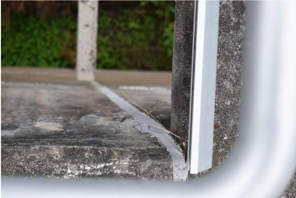
Photo 43 – Expansion Joint at North Wall of Basin No. 1
