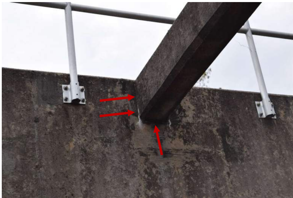
Photo 46 – Connection of North Wall of Basin No. 1 to East Bracing Strut Punching shear cracks along the perimeter of the bracing strut.
