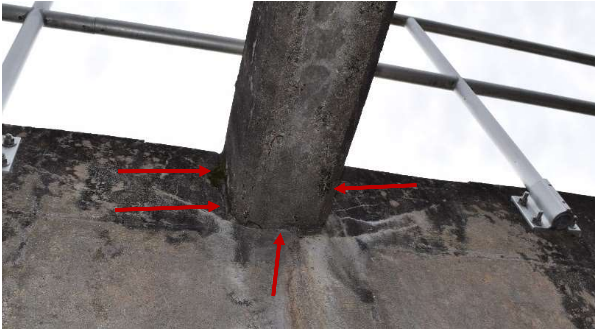
Photo 25 – South Wall of Basin No. 2 at West Bracing Strut – (Looking South) Punch-trough failure of the strut at the connection with the wall.
