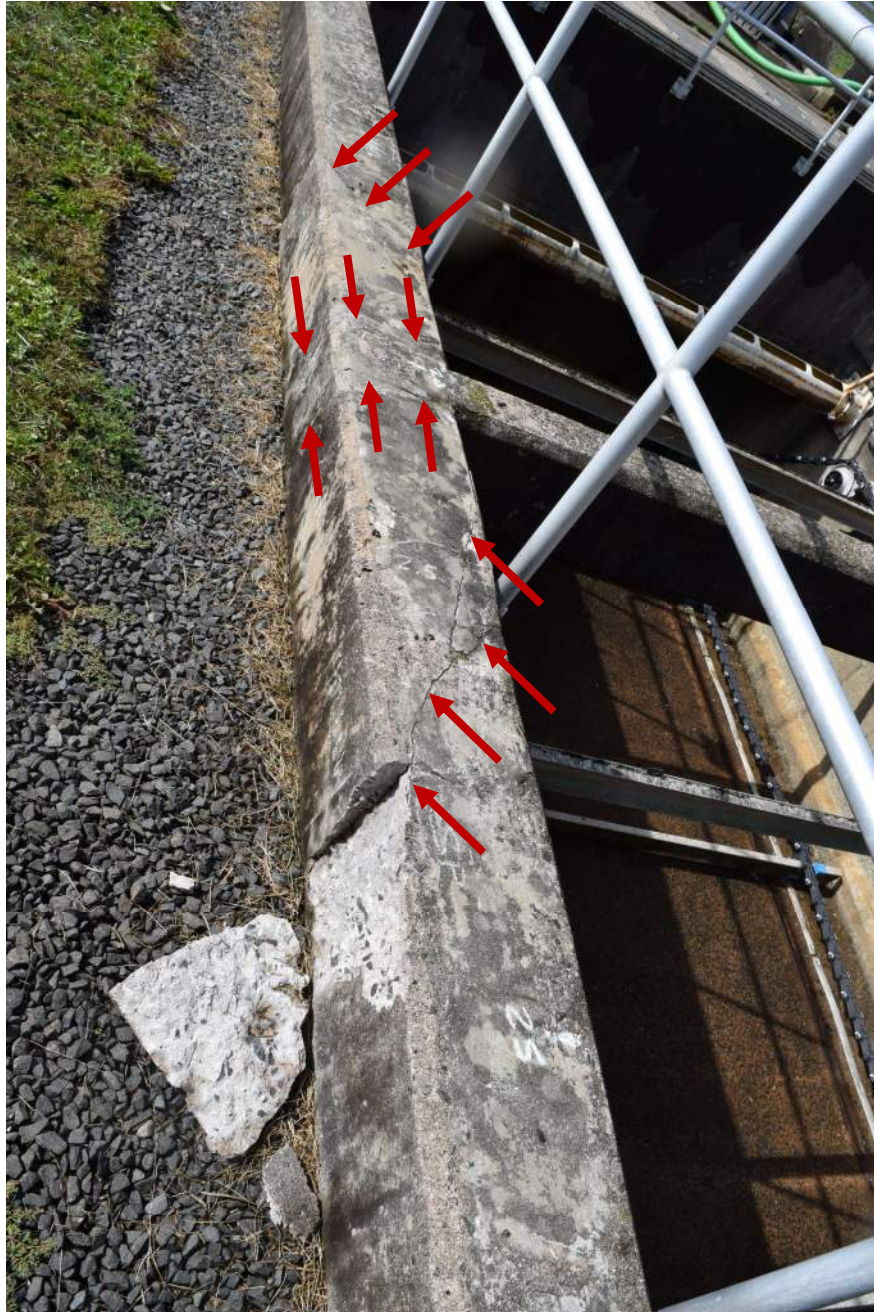
Photo 7 – South Wall of Basin No. 2 at West Bracing Strut (Looking West) Shear cracks in the South Wall of Basin No. 2 on each side of the West Bracing Strut, and punching shear cracks along the perimeter of the Bracing Strut.
