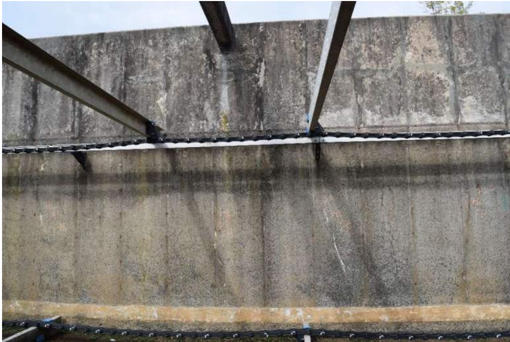
Photo 32 – Center Wall of Basin No. 2 at East Bracing Strut – (Looking North) General view of the connection between the East Strut and the Center Wall of Basin No. 2. Slight cracking was observed at the connection of the strut to the wall.
