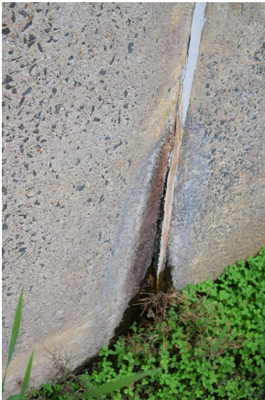
Photo 44 – Expansion Joint at North Wall of Basin No. 1
