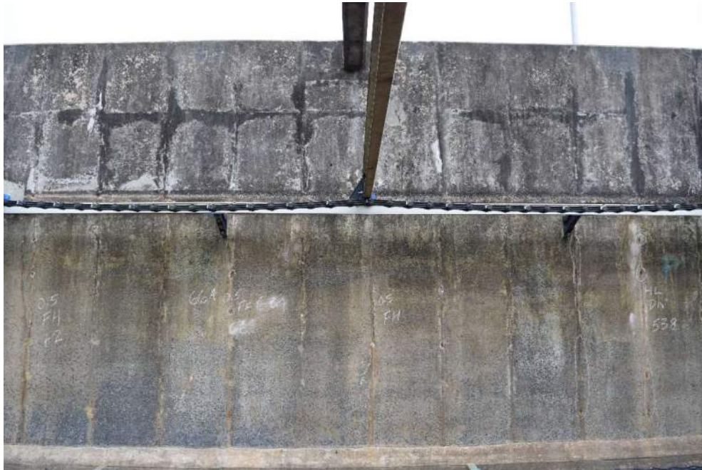
Photo 36 – Center Wall of Basin No. 1 at East Bracing Strut – (Looking South) General view of the connection between the East Strut and the Center Wall of Basin No. 1. Slight cracking was observed at the connection of the strut to the wall.
