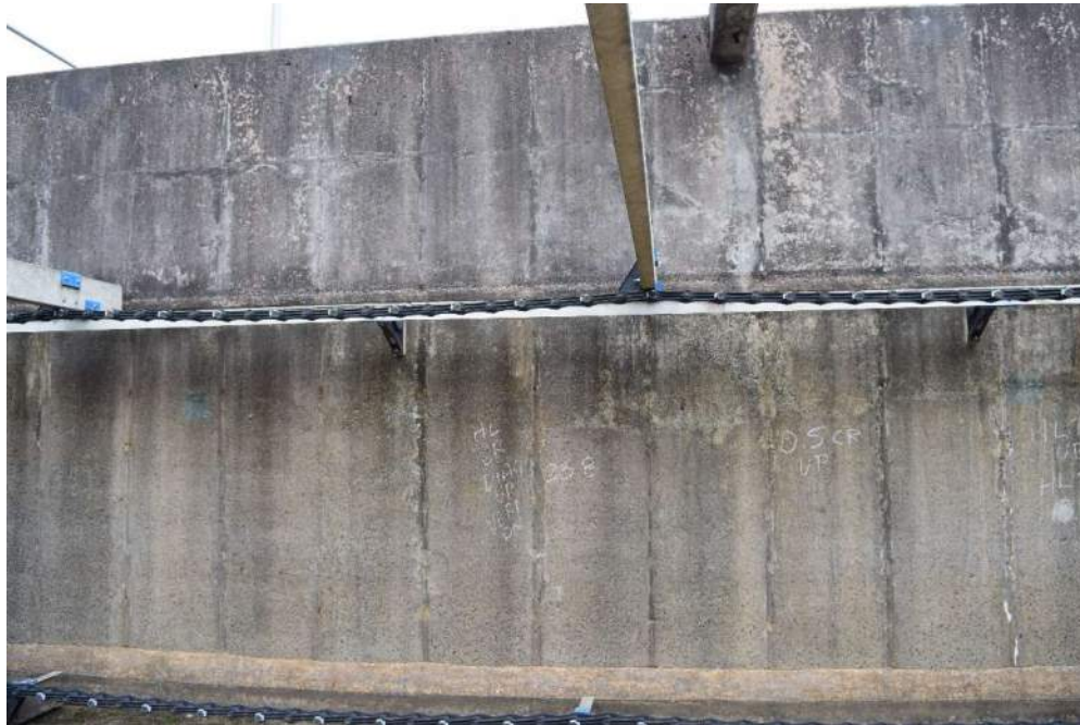
Photo 34 – Center Wall of Basin No. 1 at West Bracing Strut – (Looking South) General view of the connection between the West Strut and the Center Wall of Basin No. 1. Slight cracking was observed at the connection of the strut to the wall.
