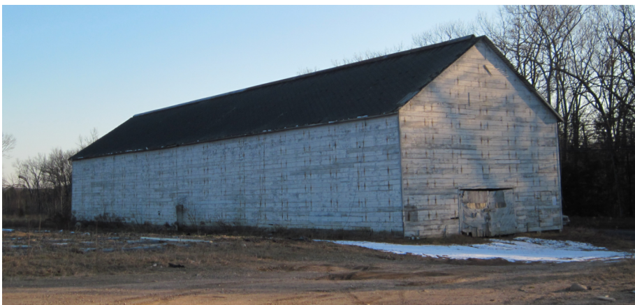
Tobacco barn, horizontal hinge ventilating system, Hoskins Rd.
