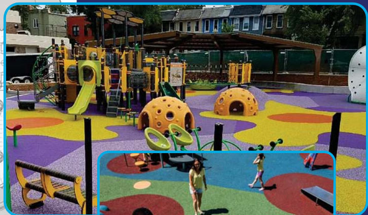
4 SITE WORK POURED-IN-PLACE SURFACE @ PLAYSAPES
