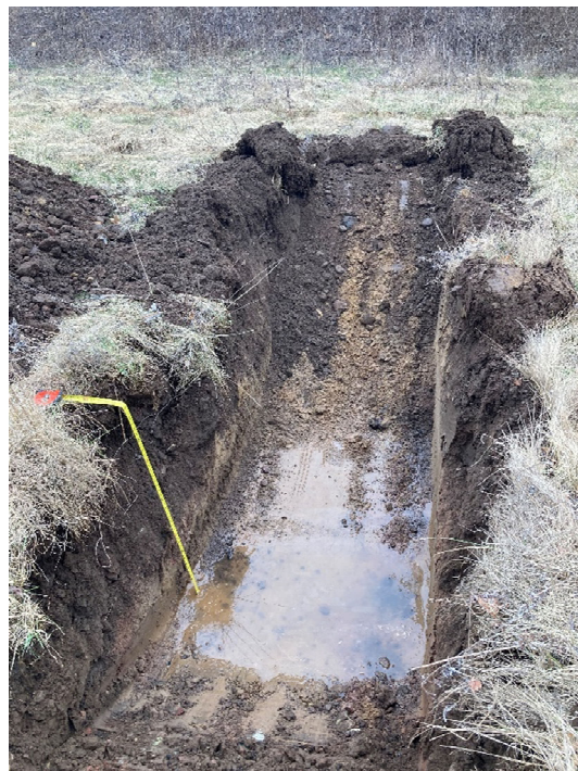
Test Pit 2 at 9:25 am on March 31, 2021
