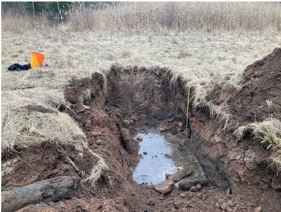
Test Pit 4 at 9:47 am on March 31, 2021
