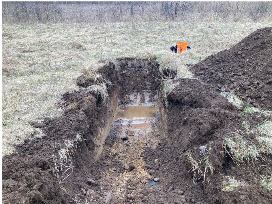
Test Pit 3 at 9:35 am on March 31, 2021
