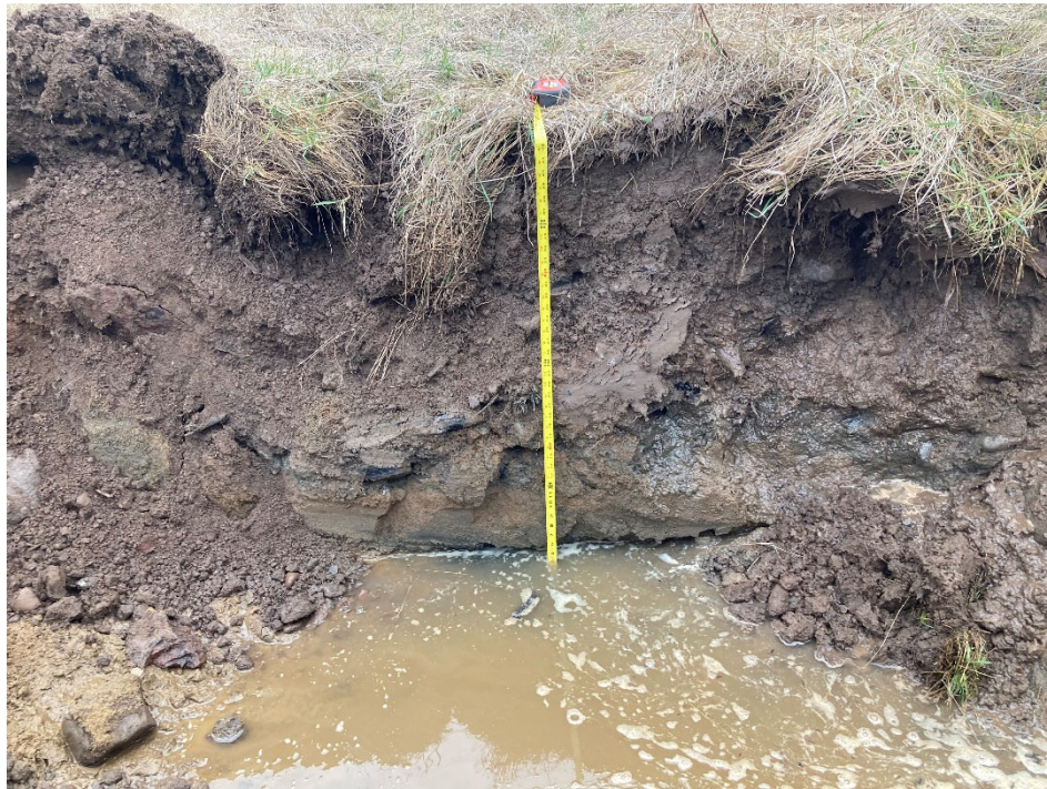
Test Pit 3 at 9:33 am on March 31, 2021
