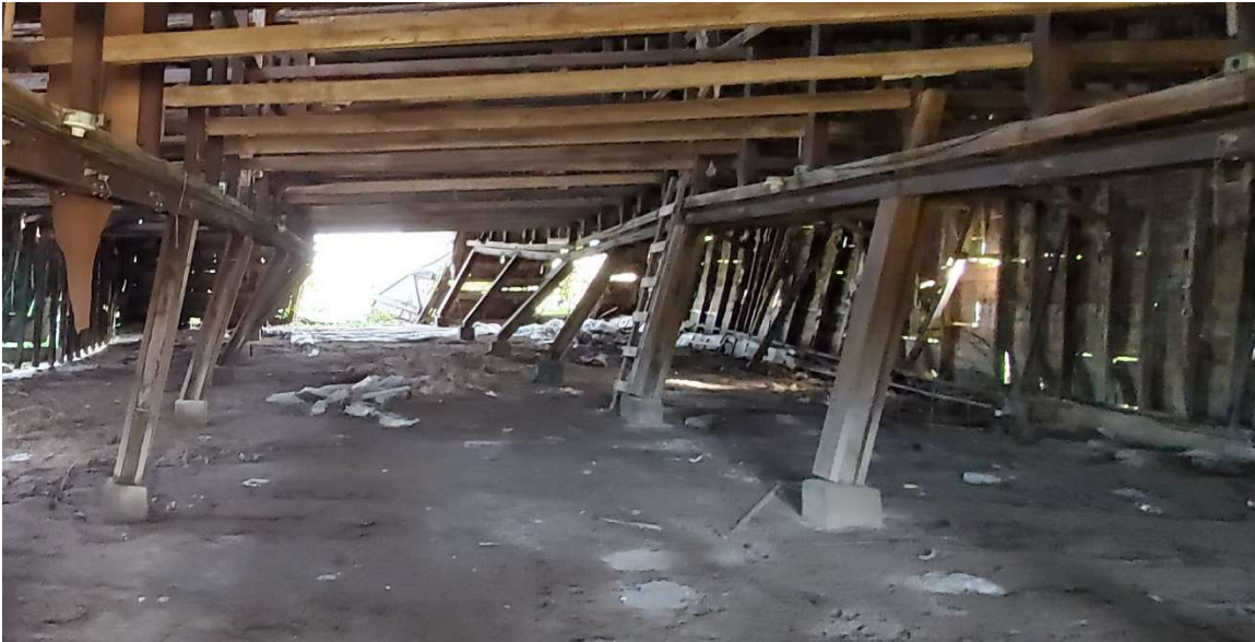
Photo No. 3 Barn No. 1 – Enlarged View of partial collapse of Barn Framing System (Center and East Bay)
