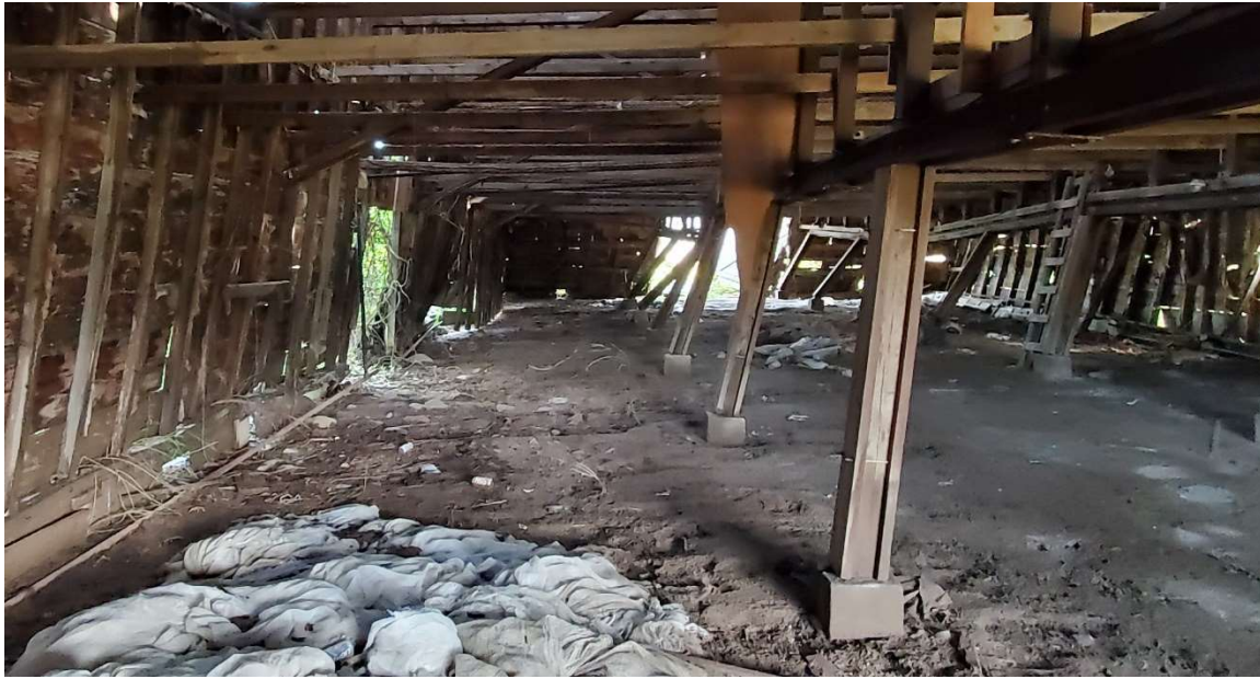
Photo No. 5 Barn No. 1 – Enlarged View of partial collapse of Barn Framing System (West and Center Bays)
