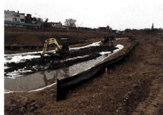
Structural Project (stream daylighting)
