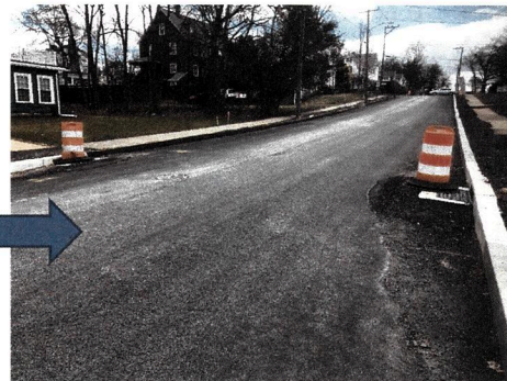
Hart Street Drainage System Project Photo by David Murphy, 2018
