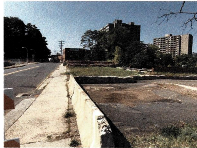
Removal of Structures from Floodplain
