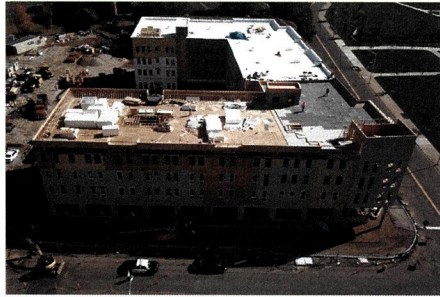
New Elevated Construction
