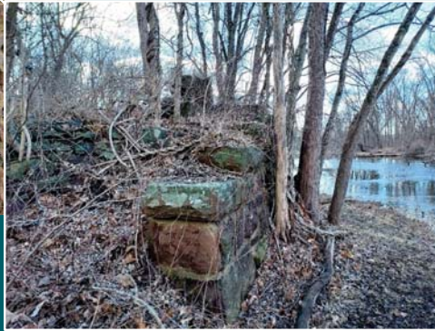
Historic rail bridge abutment
