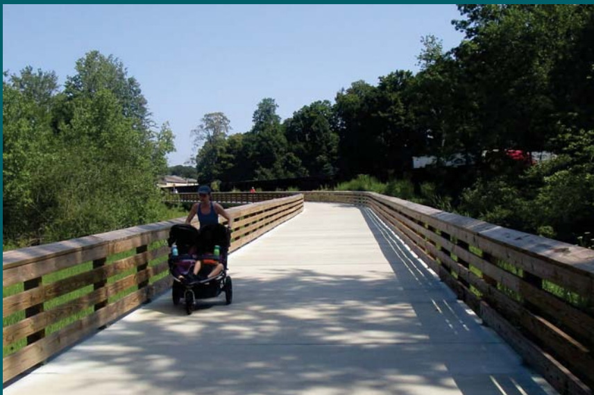
Example of CTDOT-built boardwalk trail in Cheshire
