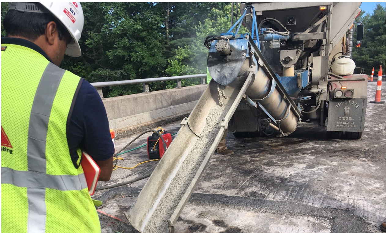
Drake Hill Road Bridge Construction
