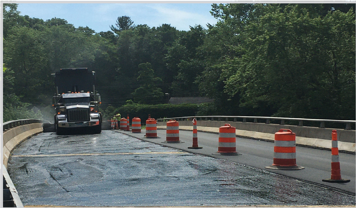
Drake Hill Road Bridge Rehabilitation
