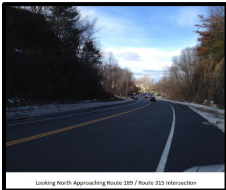
Looking North Approaching Route 189 / Route 315 Intersection
