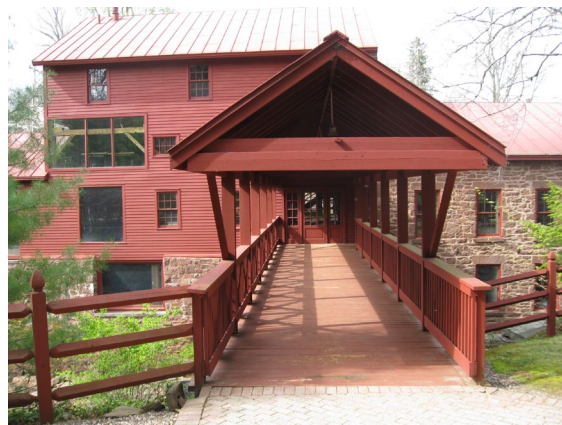
Existing bridge structure from 1980s
