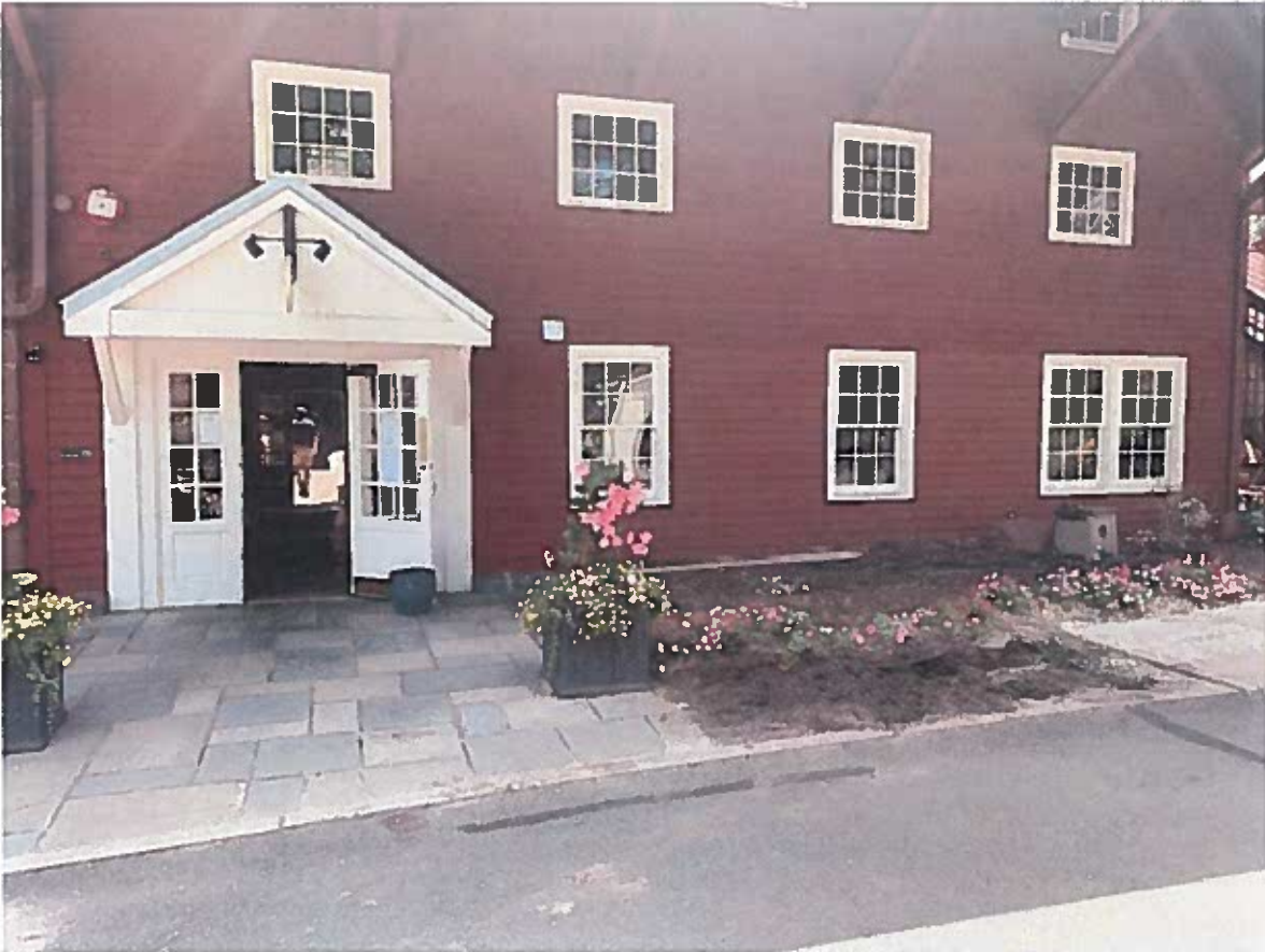
Millwrights existing entrance 10/1/2023
