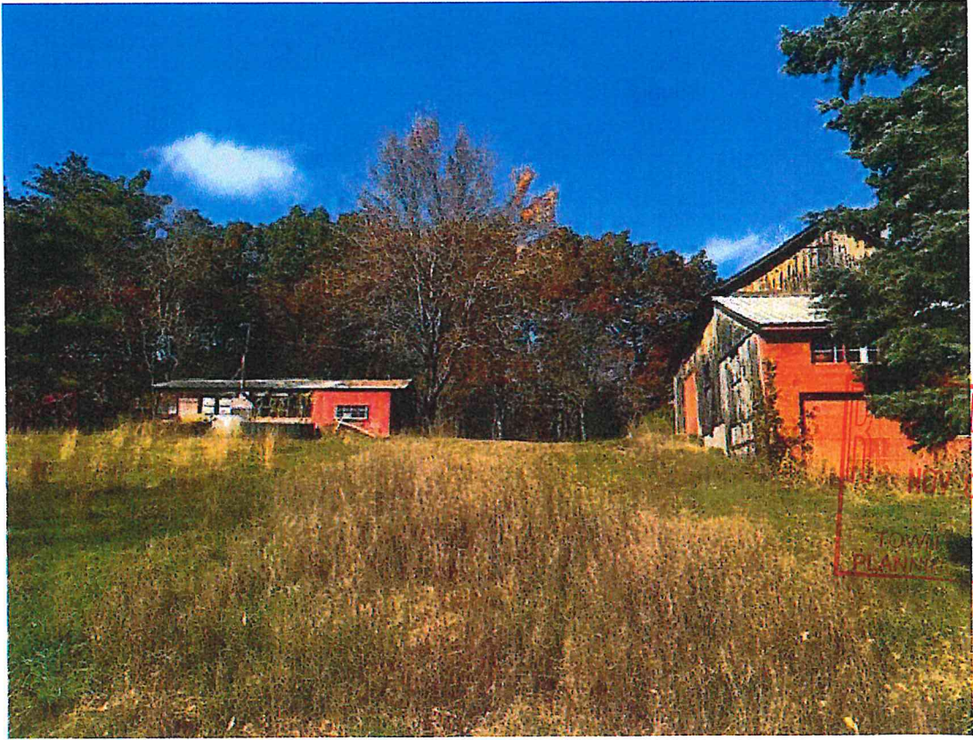
View looking up at front shed to be removed
