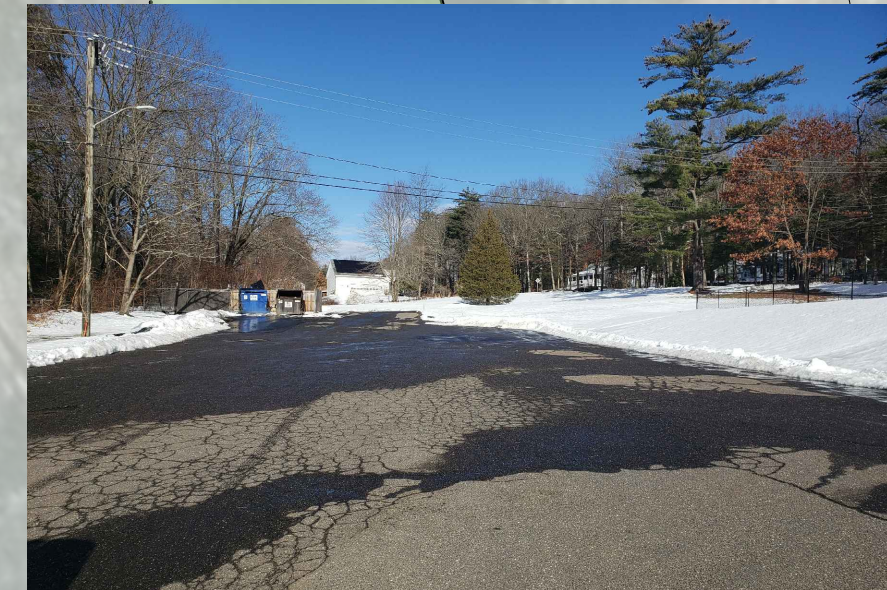
Existing Parking Lot / View To North
