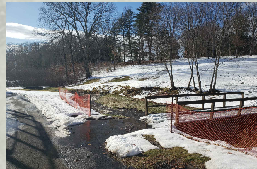
Existing Stream Crossing
