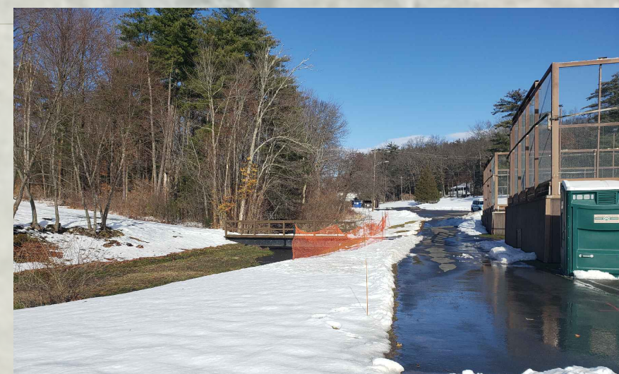
Existing Grass Wetland & Stream Looking North
