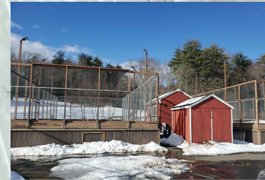
Existing Access To Court 2
