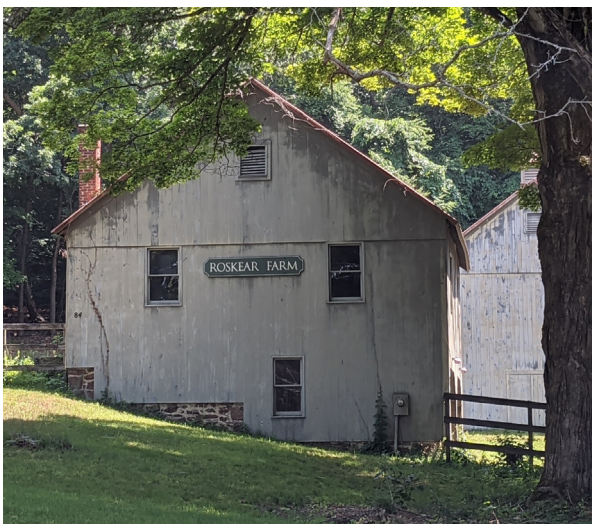
1927 Barn at Roskear Farm, 84 East Weatogue Street.
