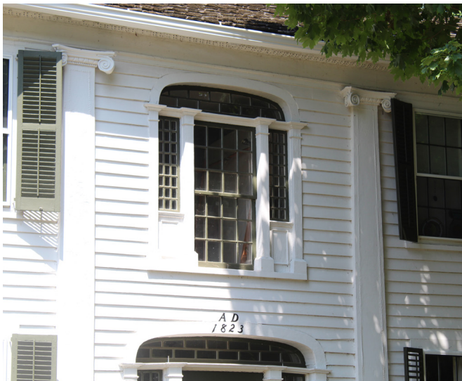
Example of a home in the District with 12 over 12 windows and columns. Source: FHI Studio.
