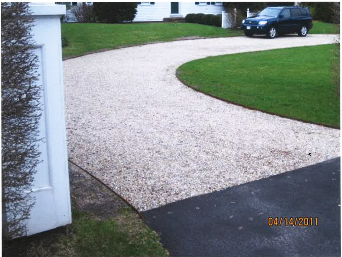
Tan and Chip driveway with Asphalt Apron (14 ft.)
