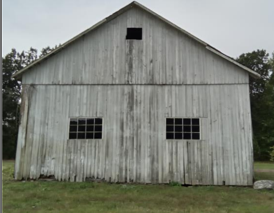
24" x 24" Window (Missing) – Left Side of Barn on the Upper Level
