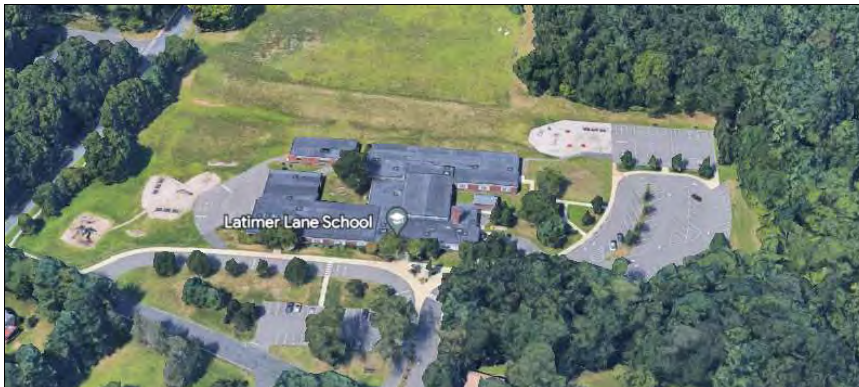
Latimer Lane School Renovation
