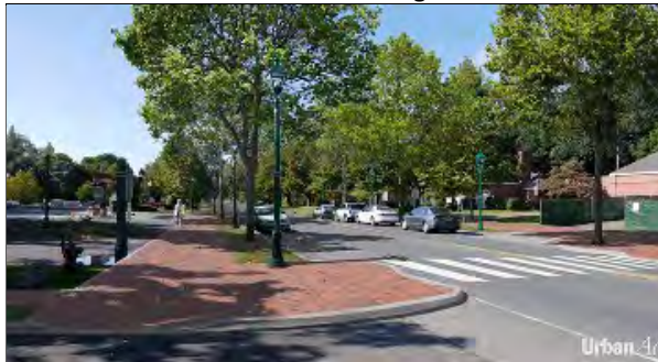
Removal of overhead wires. addition of brick sidewalks and “bumpouts” to narrow travel lanes, addition of crosswalks, streetlights, street trees, and on-street parking
