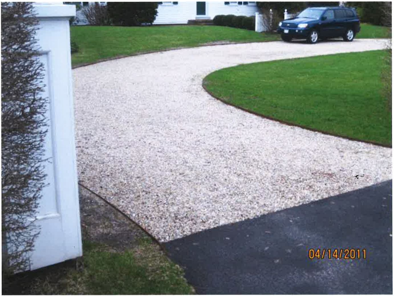
Tar and Chip driveway with Asphalt Apron (14 ft.)
