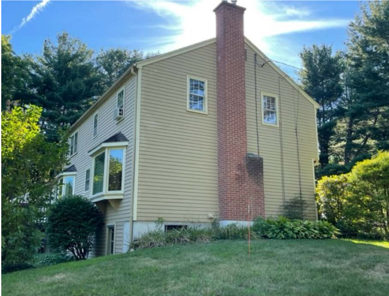
West side view (note the orange stake in foreground marks distance of the proposed one story addition from house)
