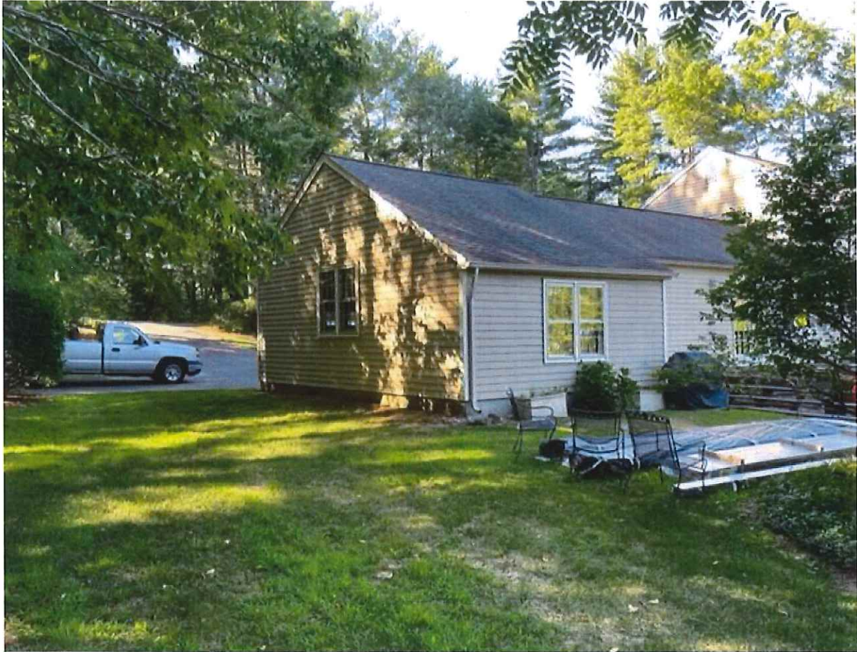
East side view (showing attached garage)
