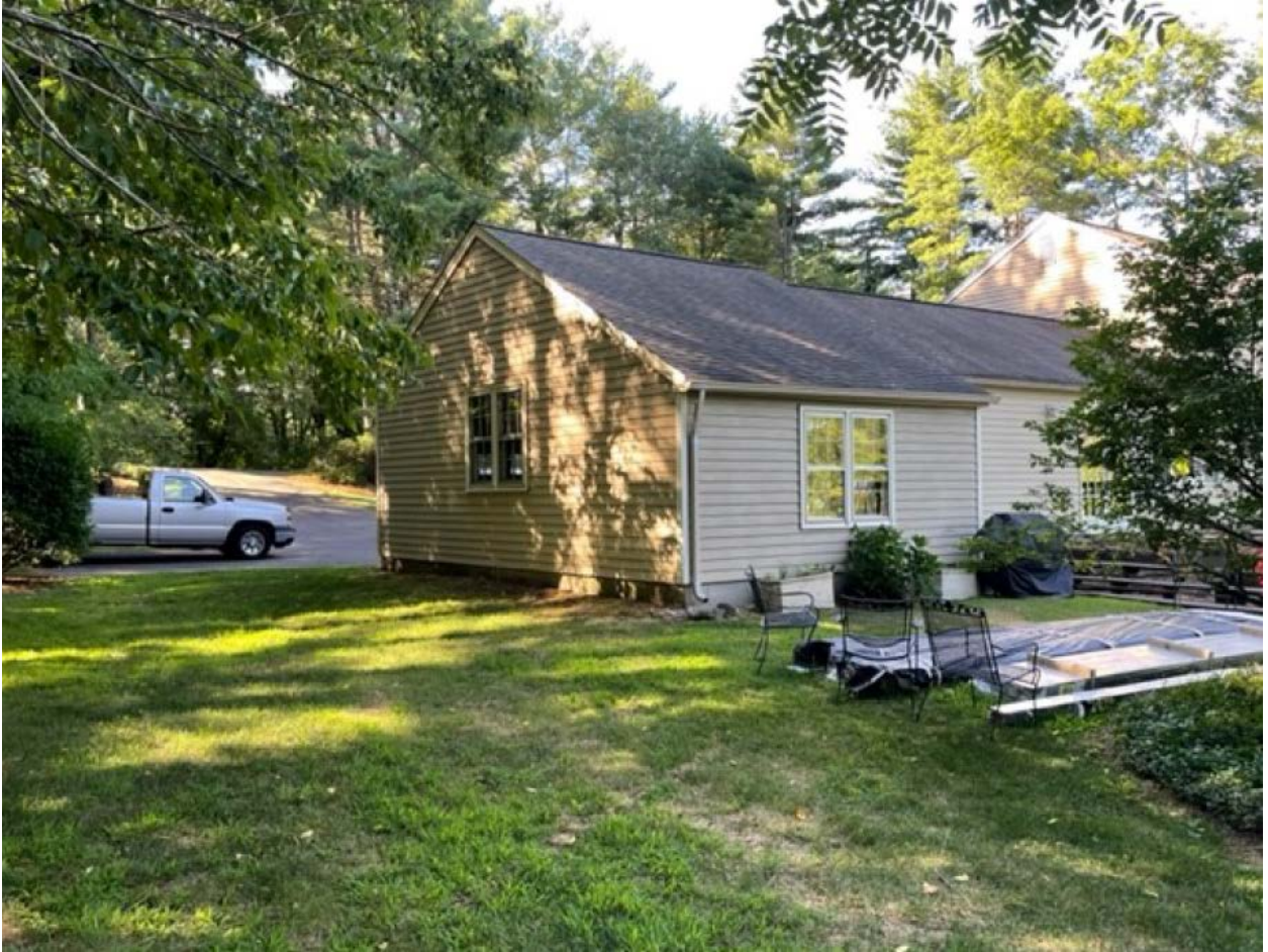
East side view (showing attached garage)
