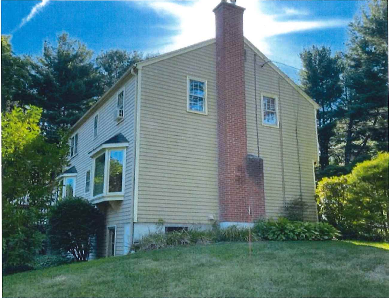
West side view (note the orange stake in foreground marks distance of the proposed one story addition from house)
