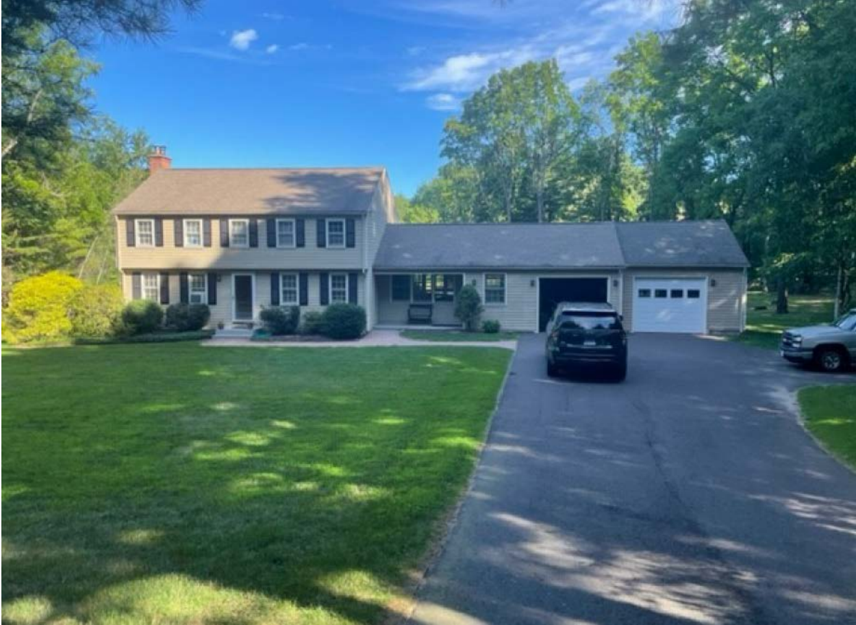
Front view (note that house faces South)
