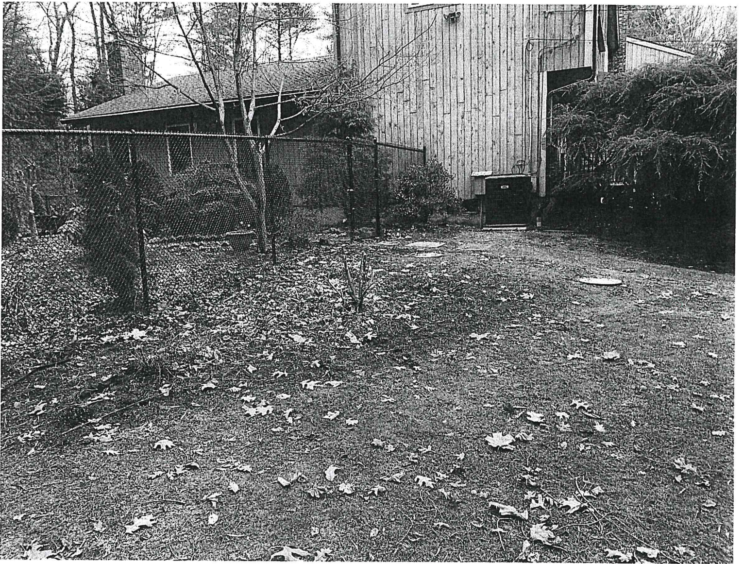
SEPTIC ACCESS LIDS + NORTH SIDE OF HOUSE
