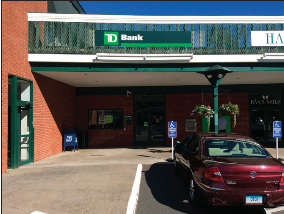
EXISTING SITE PHOTOGRAPH
