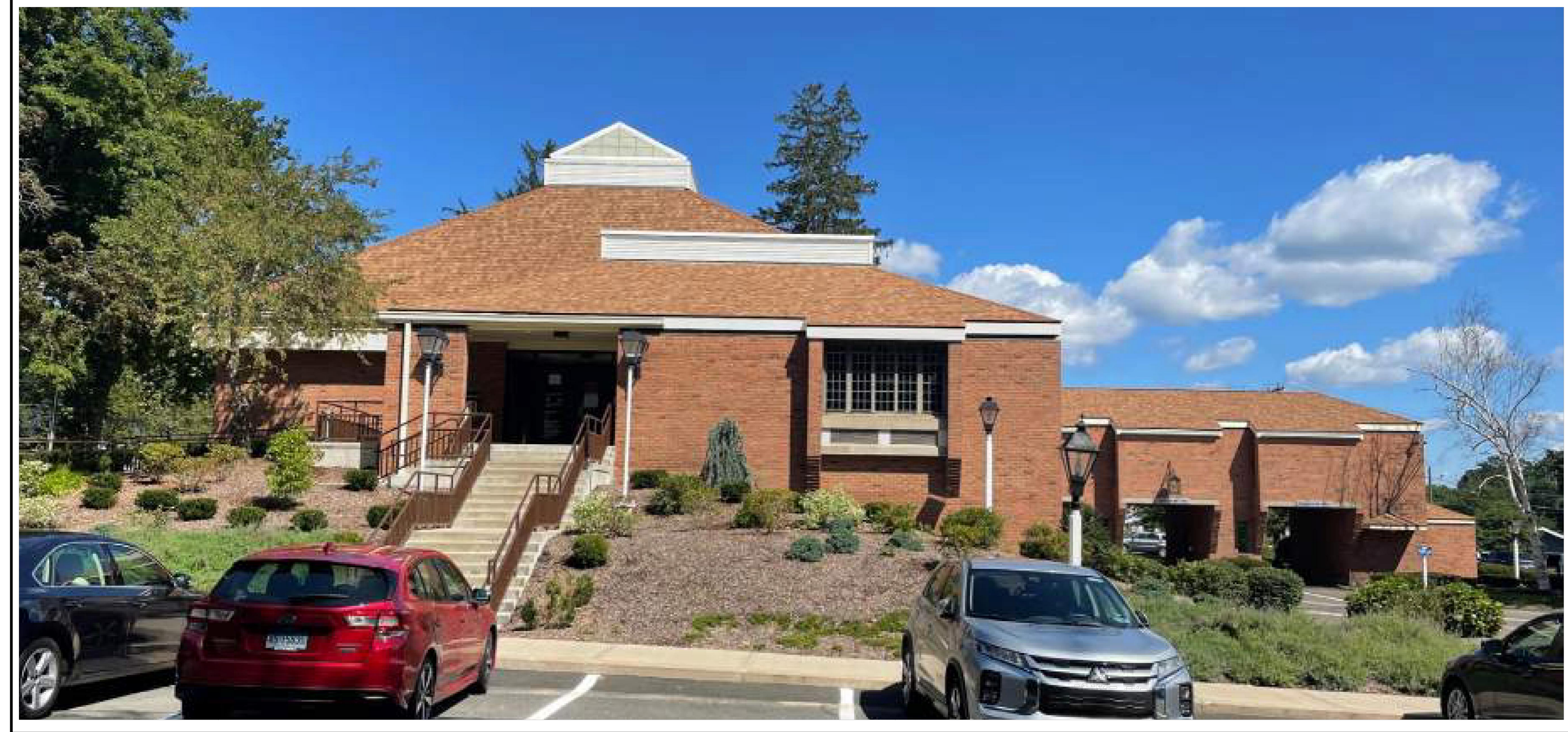
PROPOSED DESIGN AT SOUTHWEST ELEVATION (SIGNAGE INDICATED HAS BEEN APPROVED UNDER A SEPARATE PERMIT) SCALE: N.T.S. ③
