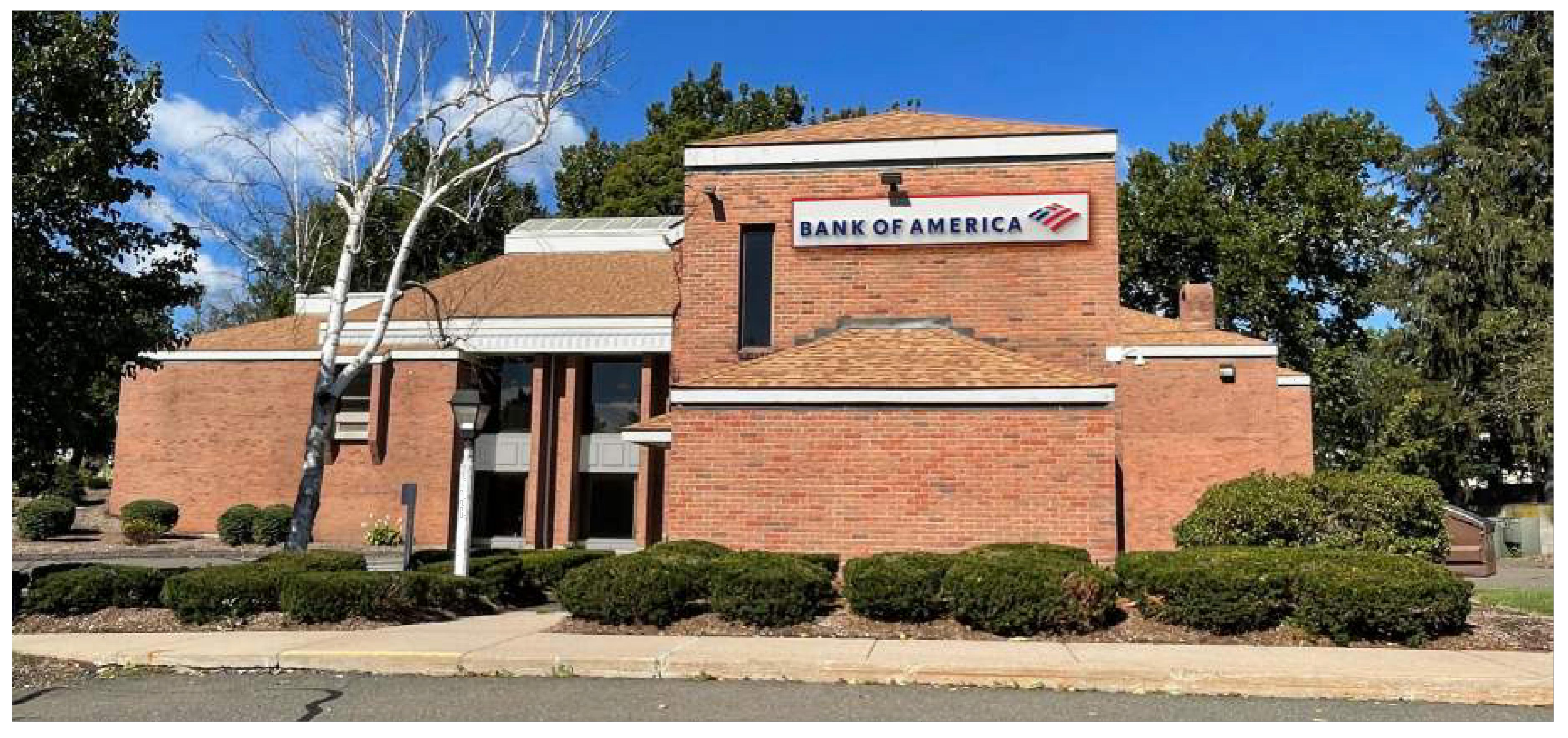
PROPOSED DESIGN AT SOUTHEAST ELEVATION (SIGNAGE INDICATED HAS BEEN APPROVED UNDER A SEPARATE PERMIT) SCALE: N.T.S. ②
