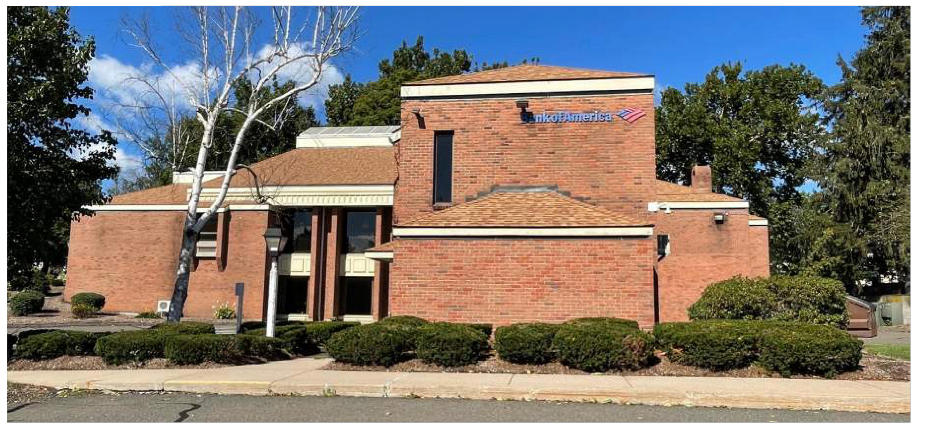
EXISTING CONDITIONS AT SOUTHEAST ELEVATION SCALE: N.T.S. ②
