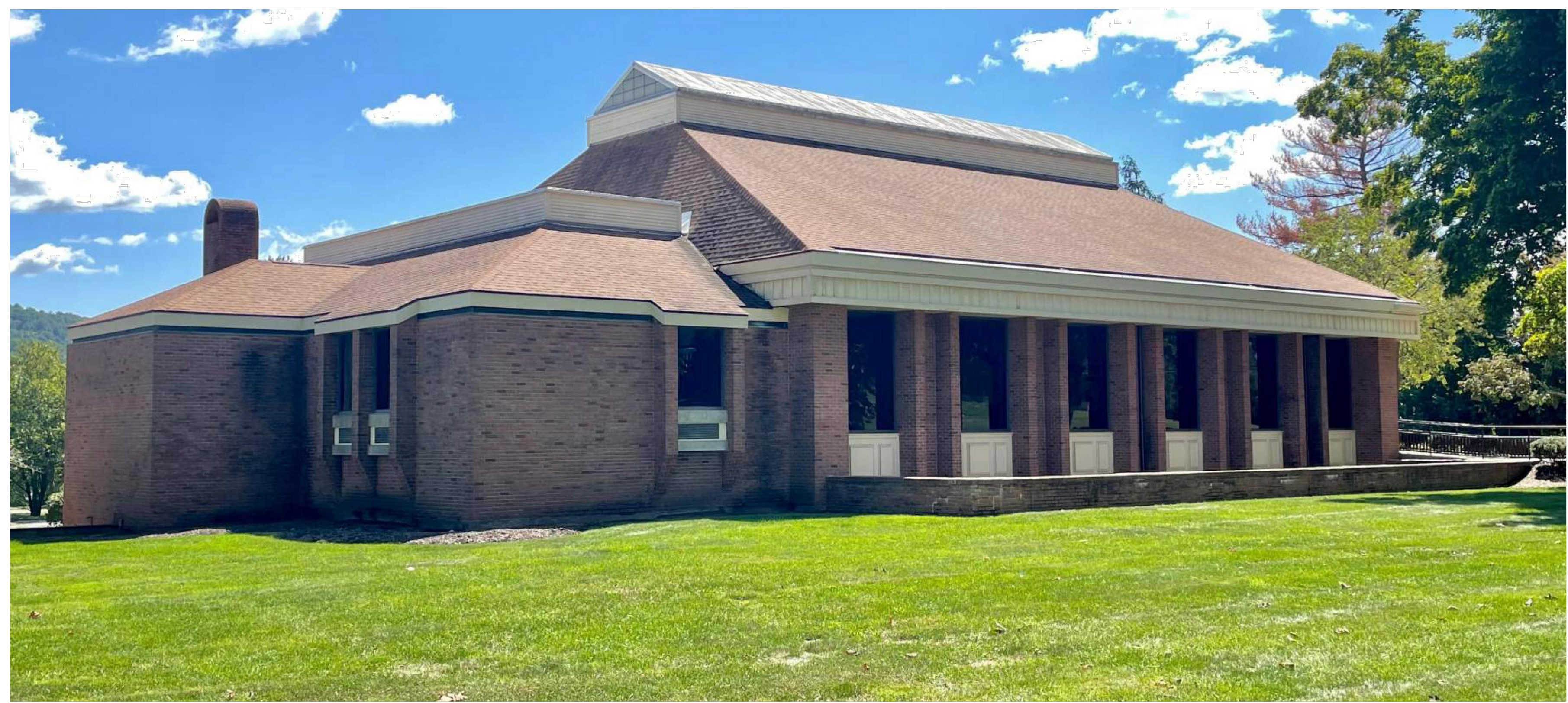
EXISTING CONDITIONS AT NORTHWEST CORNER SCALE: N.T.S. ①
