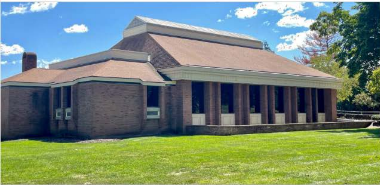
EXISTING CONDITIONS AT NORTHWEST CORNER SCALE: N.T.S. ①
