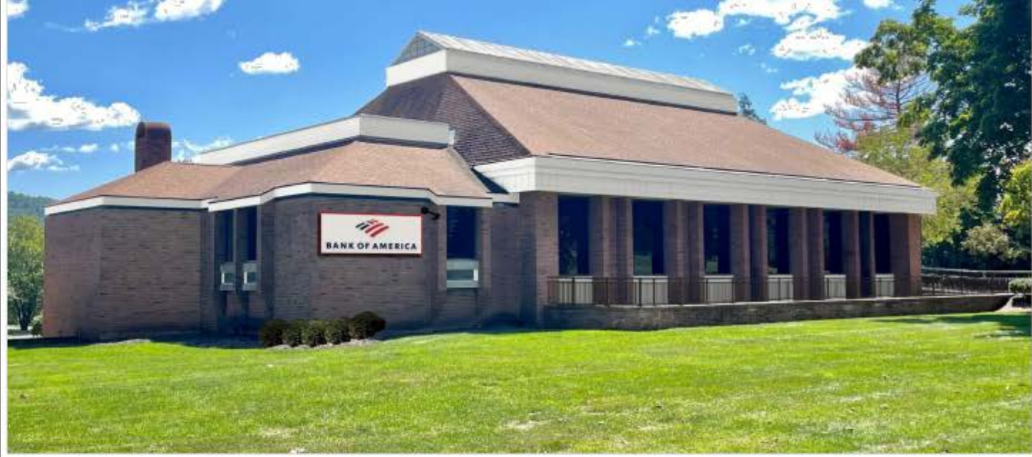
PROPOSED DESIGN AT NORTHWEST CORNER (SIGNAGE INDICATED HAS BEEN APPROVED UNDER A SEPARATE PERMIT) SCALE: N.T.S. ①
