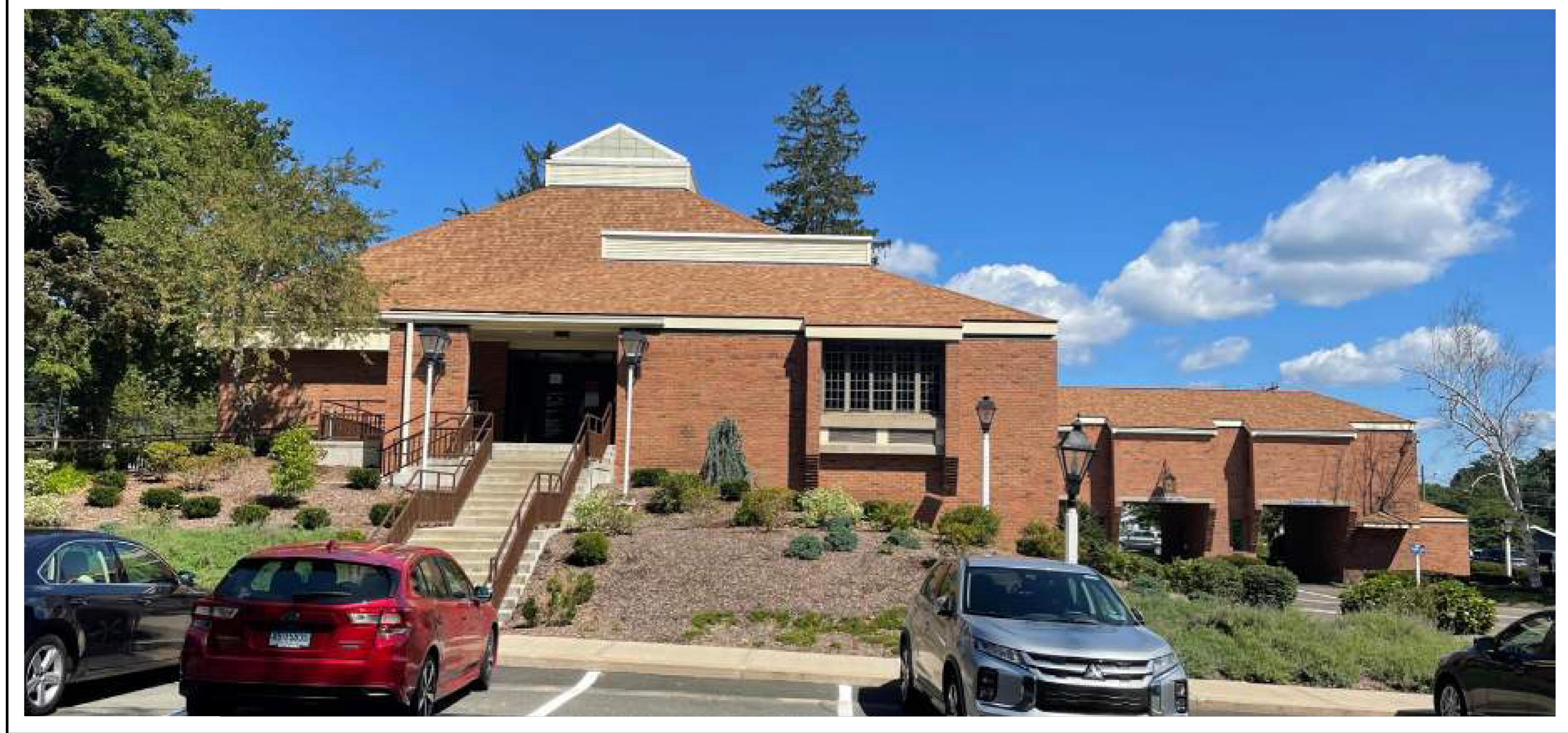
EXISTING CONDITIONS AT SOUTHWEST ELEVATION SCALE: N.T.S. ③
