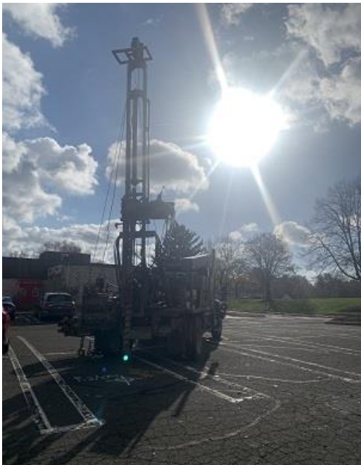
Figure 3: Drill rig setup at P-2/IF-1
