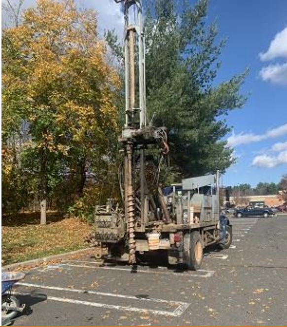
Figure 1: Offset at P-1 because of underground utility
