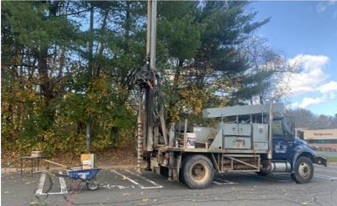
Figure 5: Drill rig setup at B-1
