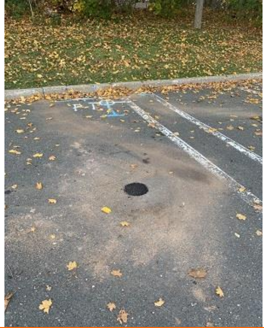
Figure 2: Example of backfilled borehole at completion
