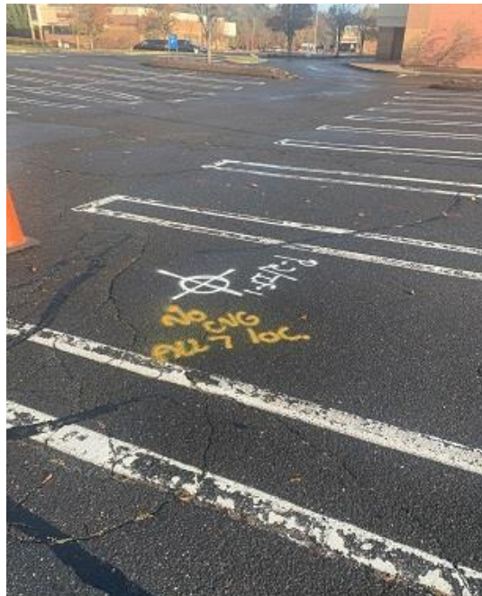
Figure 4: Example of cleared utilities
