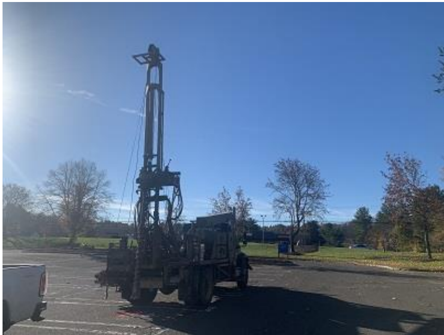
Figure 6: Drill rig setup at B-2
