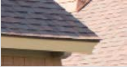
Asphalt Shingles- Brown to Match Pavilion
