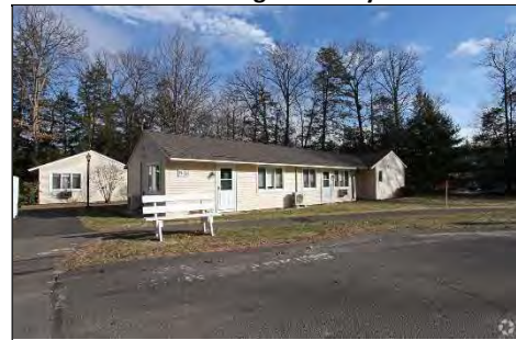
Current Housing Authority Units
