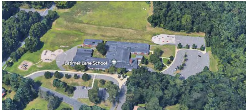
Latimer Lane School Renovation
