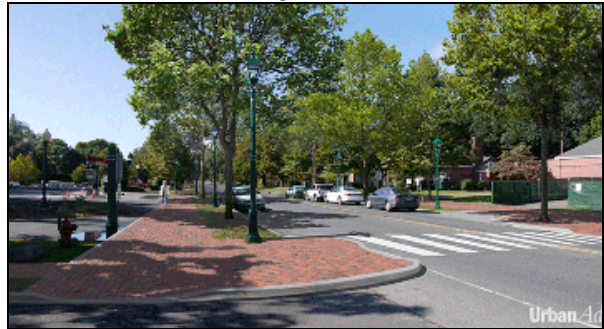
Completion of brick sidewalks plus addition of streetlights, street trees, and on-street parking
