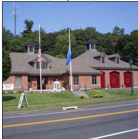
Main Fire Station (Taxing District)
