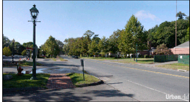
Removal of overhead wires
